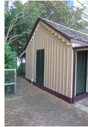
Figure 3. 28: North elevation of cottage.
