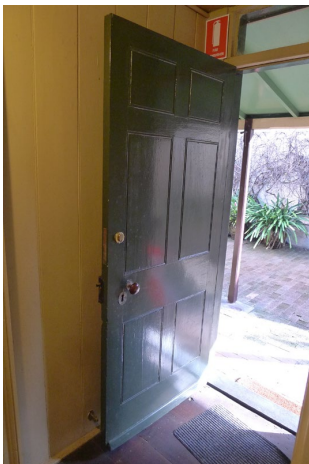
Figure 3. 72: Front door D01
