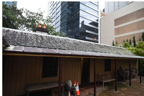
Figure 3. 25: Rear (west) elevation
