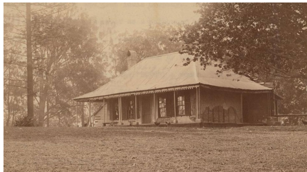
Figure 2. 5: Wollstonecraft's Crow's Nest Cottage, built in about 1821 and photographed here in the 1880s. Source: State Library of NSW (SPF/387)
