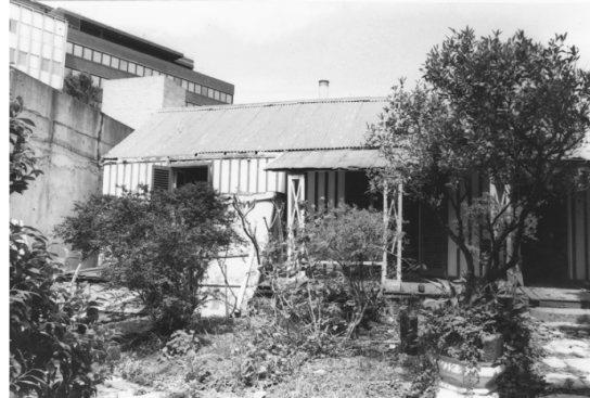
Figure 2. 41: Southern end of the front elevation of Don Bank prior to restoration works in c.1975. Courtesy: G. Britton
