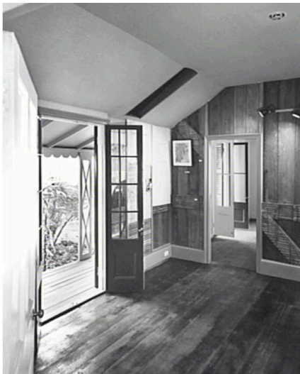
Figure 2. 48: The interior of Don Bank after completion of restoration works in 1981. Source: Stanton Library (PF 2925)
