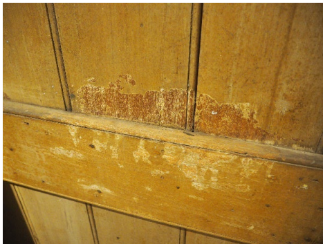
Figure 3. 70: Rail and boards in Space 05 with shiplap joints and a shaped beaded profile.
