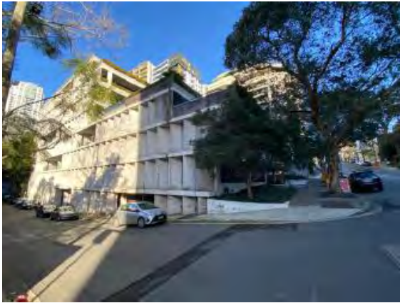
Picture 6: 41 McLaren Street illustrating the stepped nature of the building form with landscaping above
