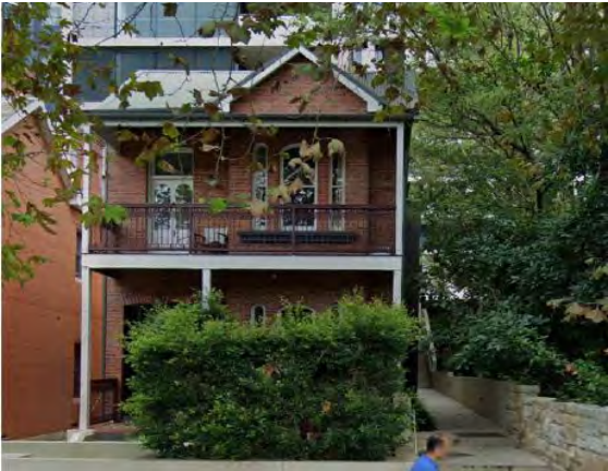
Picture 5 Heritage listed terraces at 150 Walker Street
