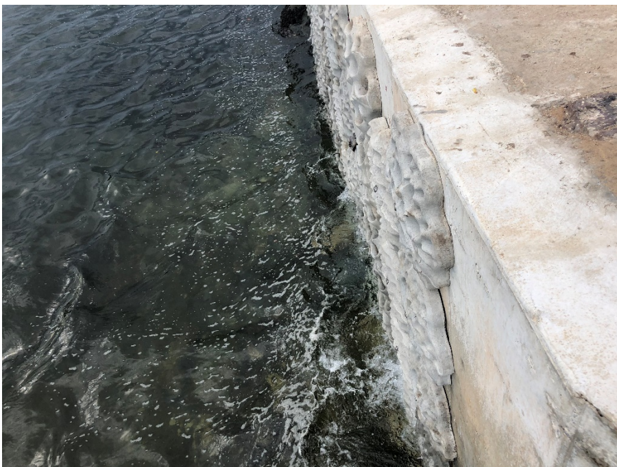
Photo 4 - Marine Habitat Tiles at Blues Point Reserve (installed January 2020)
