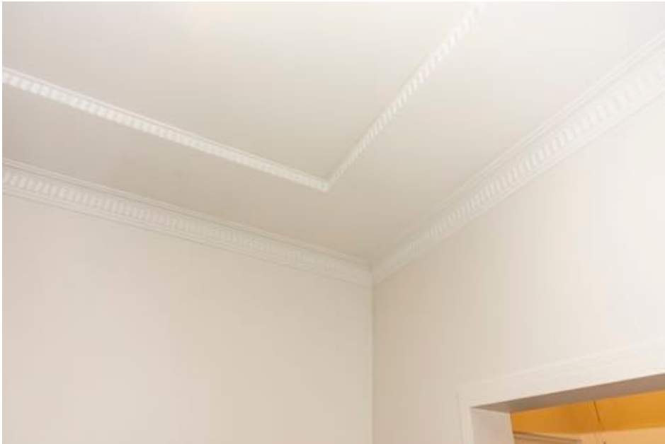
Figure 29: Unit 1 original cornice detail to ceiling in living room
