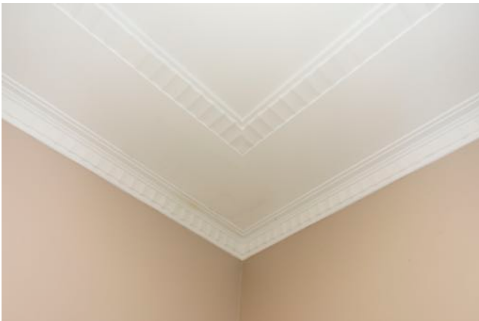
Figure 35: Cornice detail to 2 nd bedroom ceiling, Unit 1
