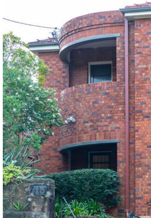
FIGURE 7: Curved corner balconies.
