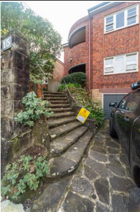
FIGURE 6: View from entry area showing tapestry brick panels to the façade and (at left) curved balconies with brick balustrades.
