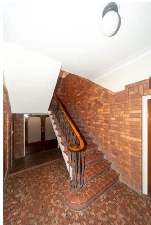
FIGURE 9: Original stairway in lobby showing original staircase, original tiling and brick and plaster wall finish.
