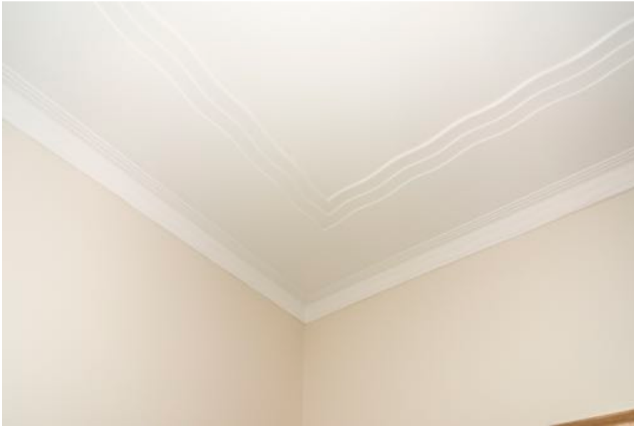
Figure 49: Unit 3 cornice detail to 2 nd bedroom
