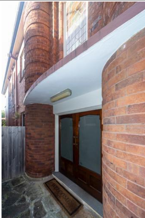
FIGURE 8: Detail around main entry doors.
