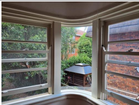
FIGURE 10: Curved glass to corner, with typical timber framed double hung windows with horizontal glazing bars to either side.
