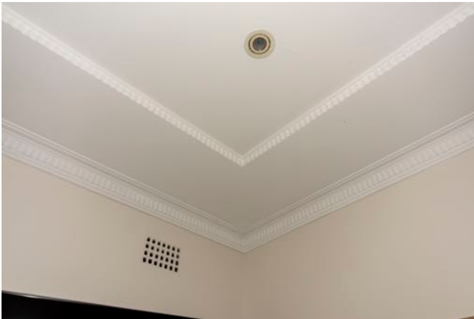
Figure 43: Original cornice to Unit 3 living room ceiling
