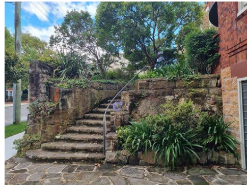
FIGURE 5: Sandstone entry steps at the site.
