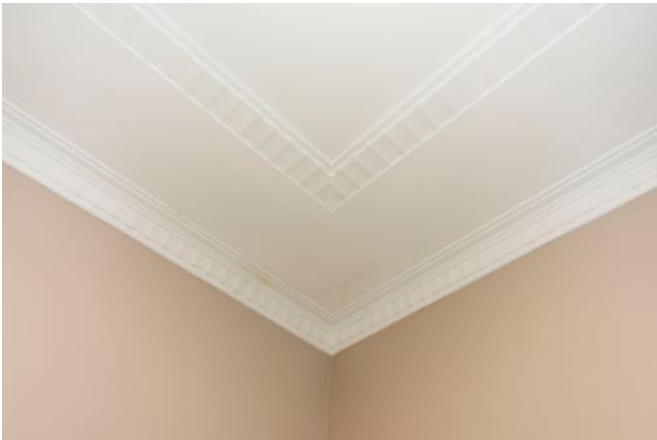
Figure 35: Cornice detail to 2 nd bedroom ceiling, Unit 1
