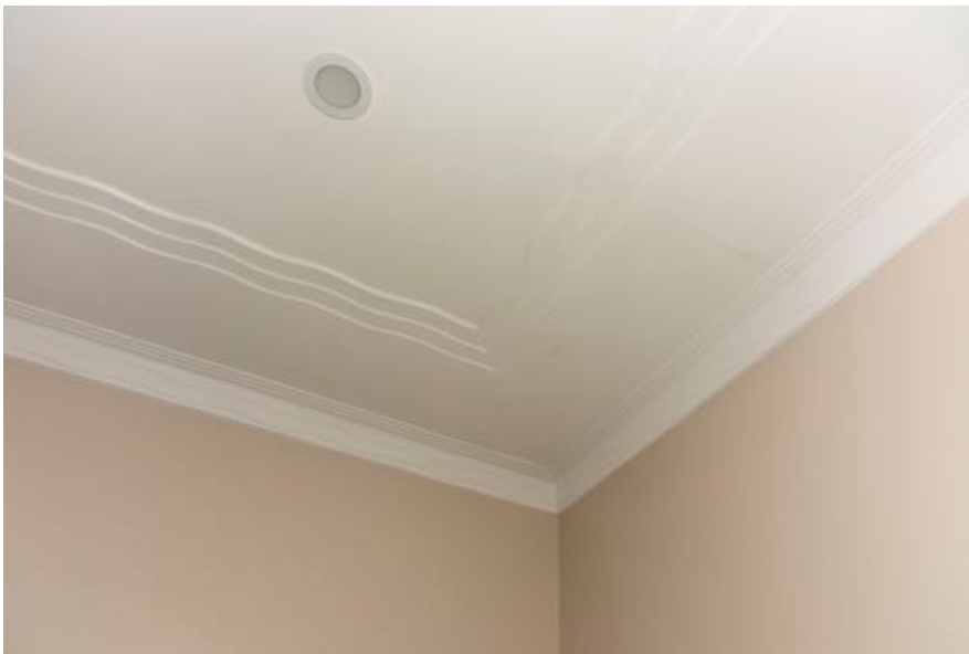
Figure 33: Original cornice detail to Unit 1 bedroom
