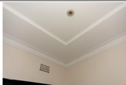
FIGURE 13: Original cornice to Unit 3 living room ceiling.
