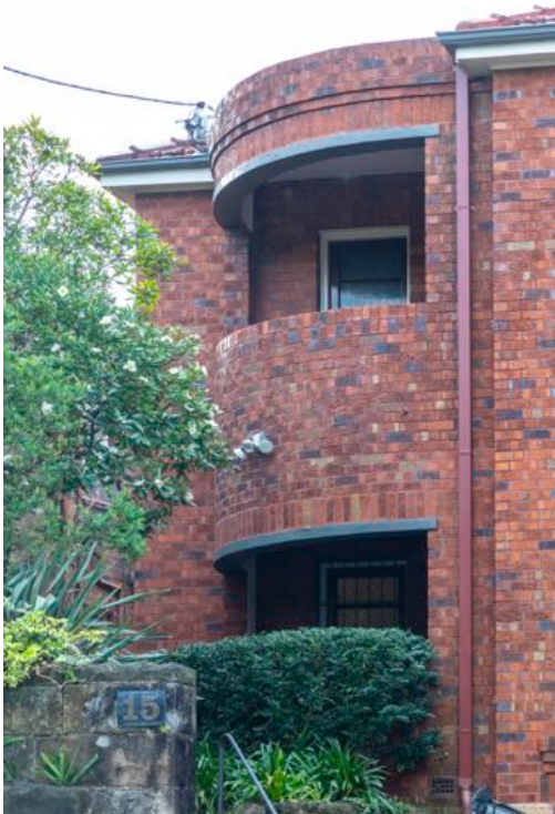
Figure 12: (Left) Curved corner balconies
