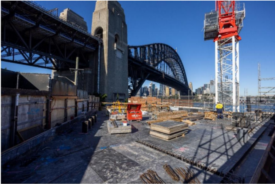
Level 4 plantroom slab formwork 29/5/2023
