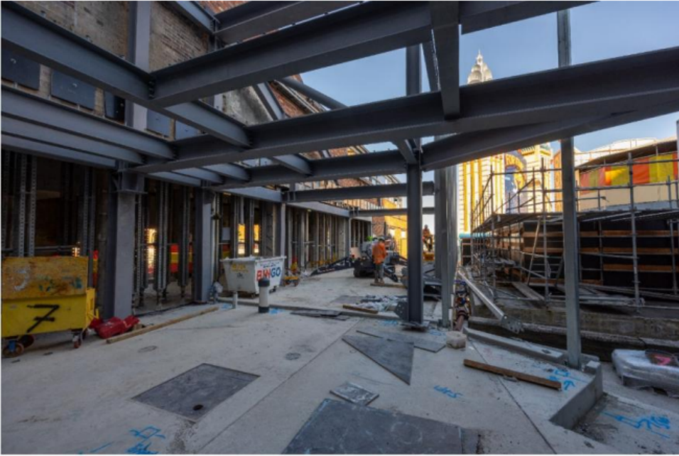
Western Stairs Steel 29/5/2023
