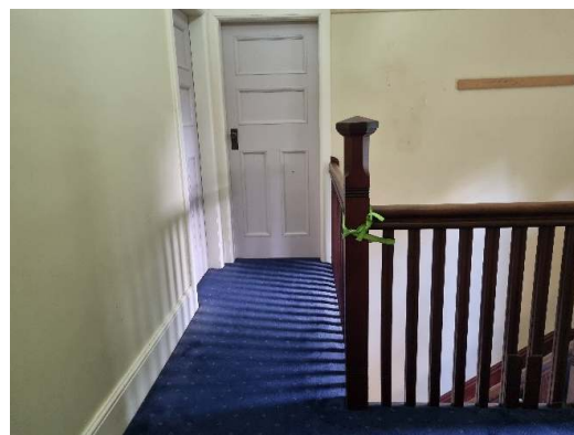
Figure 99. First floor hallway.
