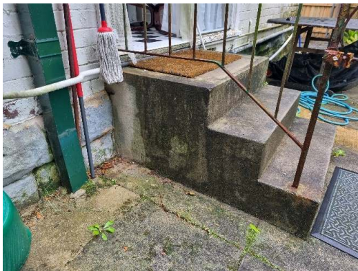
Figure 87. Stairs to rear entrance.
