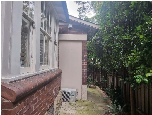
Figure 52. View along western elevation to former side entrance.
