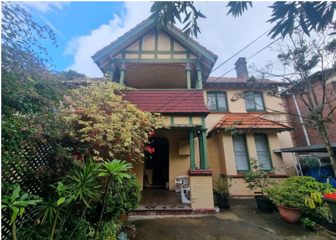
Figure 78. Front façade and entry porch.
