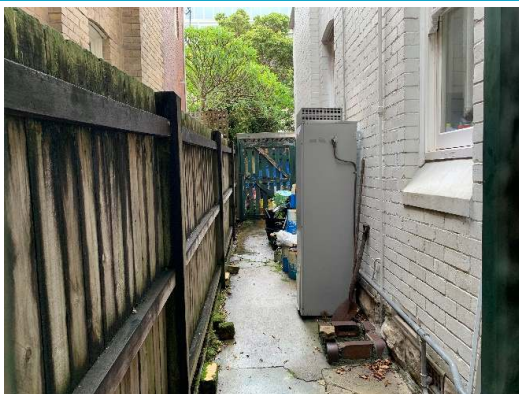
Figure 89. View along western elevation towards Yeo Street.
