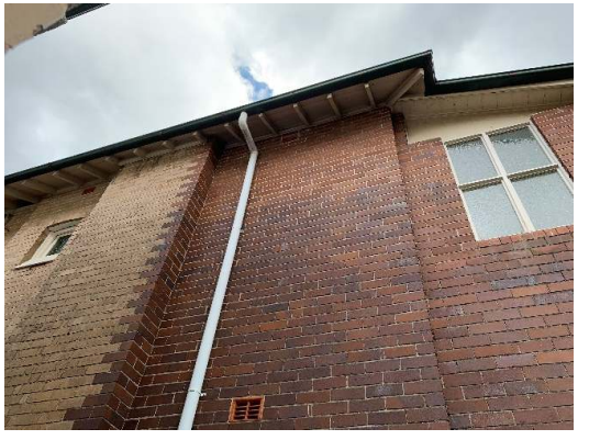
Figure 48. Eastern elevation, balcony window at right.
