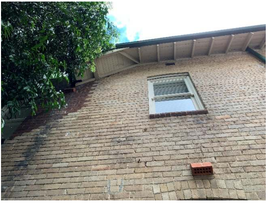
Figure 49. Eastern elevation, towards the rear of the building.
