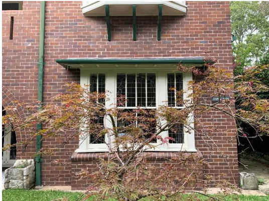
Figure 44. Ground floor window.
