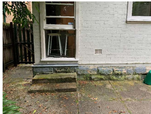
Figure 88. Stairs leading to full-length window.
