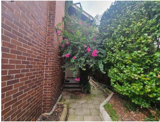
Figure 50. View to entry porch.
