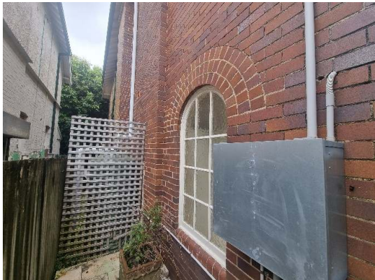
Figure 46. Eastern elevation, showing verandah window.
