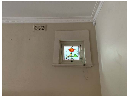
Figure 58. Feature leadlight window.
