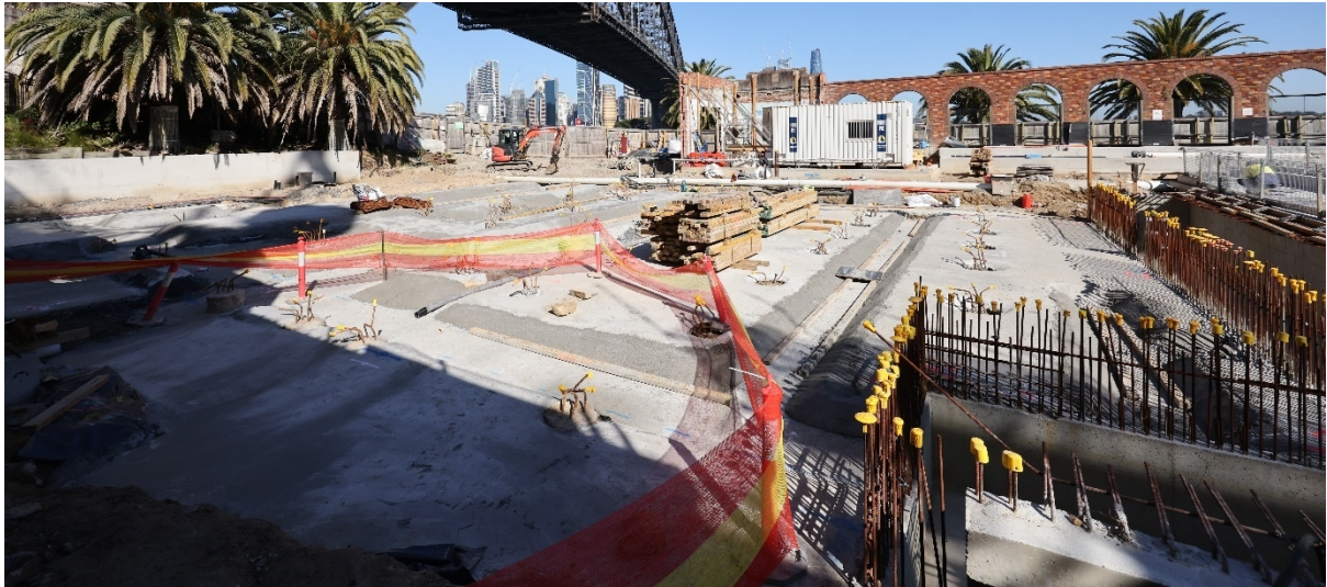
Leisure Pool blinding slab 27/7/2023
