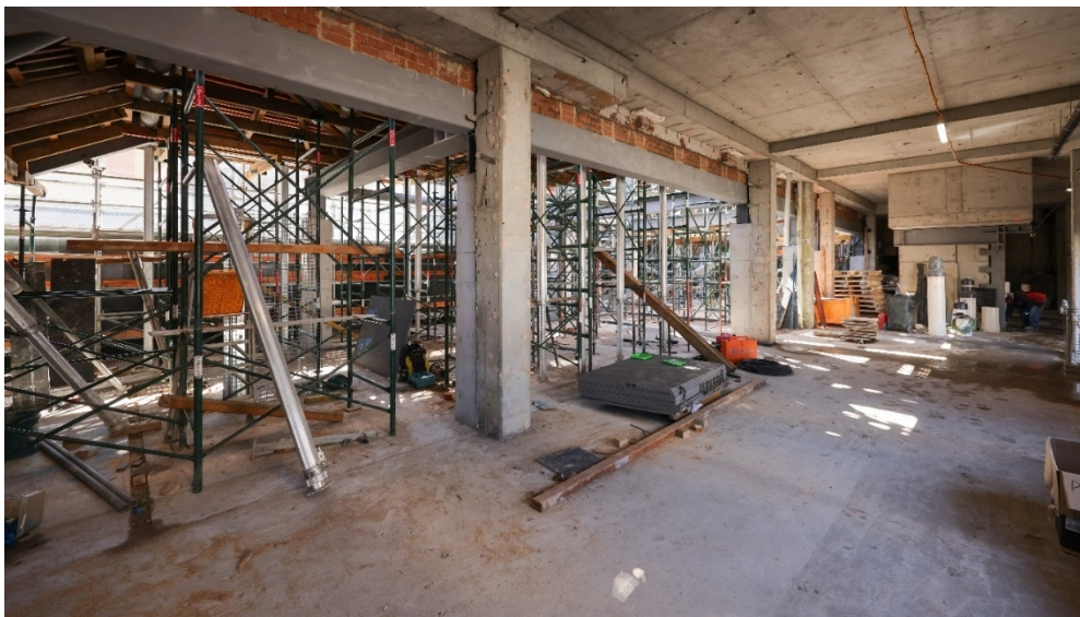
Under Western Stairs and Program Room 1 27/7/2023
