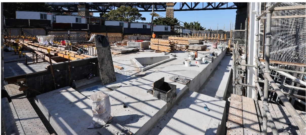
Level 4 NE plant room 27/7/2023
