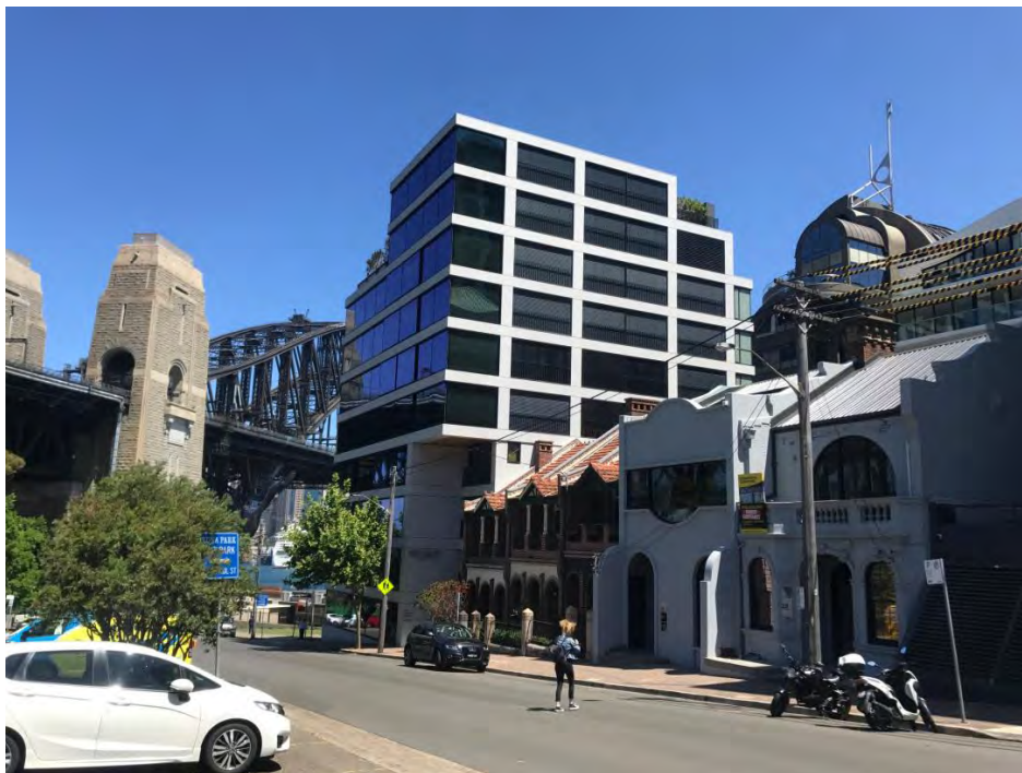
Figure 10 Residential terrace houses and building contained within 20 Alfred Street
