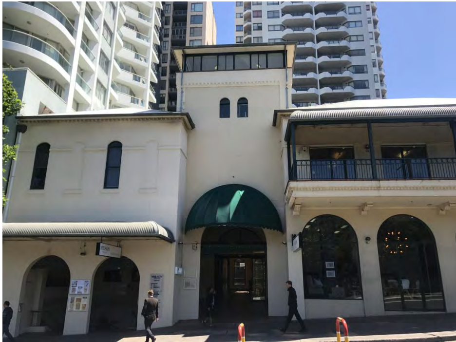
Figure 9 Adjoining building to the south
