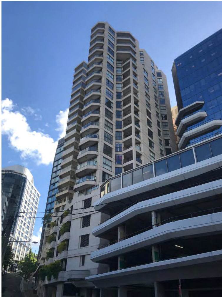
Figure 7 Adjoining building at 37 Glen Street, Milsons Point
