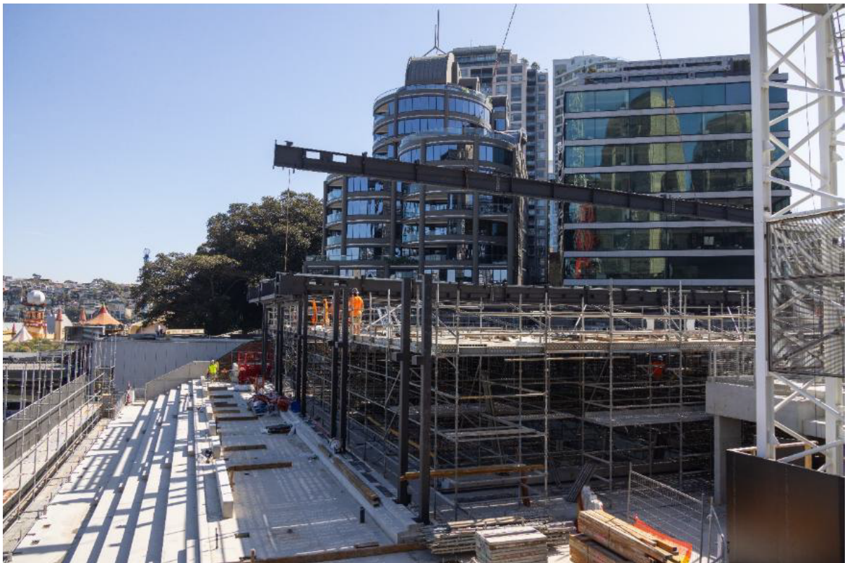
Indoor pool hall roof steel 30/8/2023
