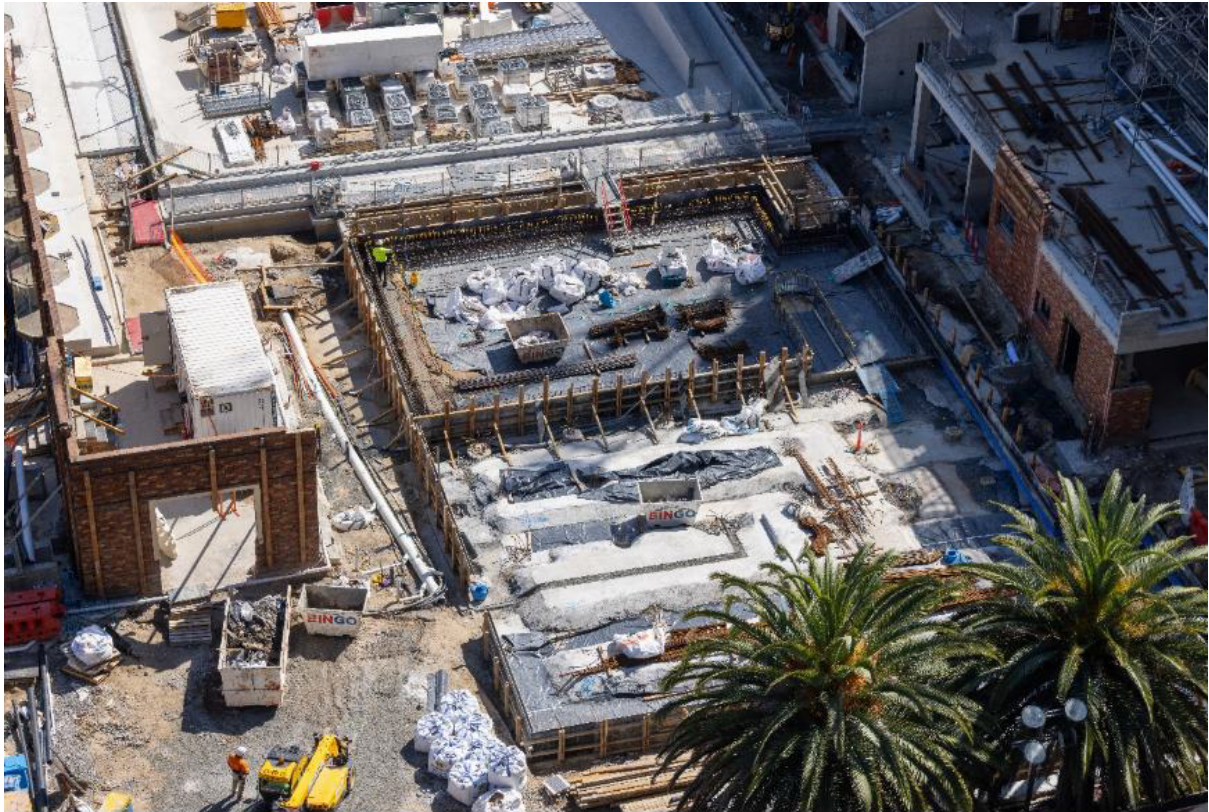
Leisure pool ready for concrete 30/8/2023
