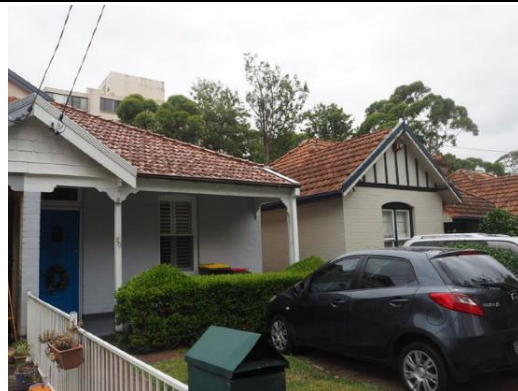
FIGURE 23: Frontage of 80 Parraween Street with No. 82 Parraween
