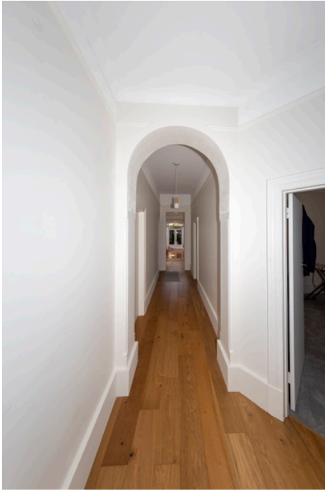
Figure 62: (Left) Central hallway looking towards the rear. Ceilings and floors are modern, The archway is early fabric, but be missing early detail.
