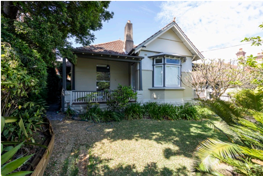
Figure 45: The front elevation of No. 9 Selwyn Street.
