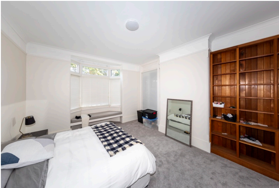
Figure 60: Front bedroom, 9 Selwyn Street, noting modern ceilings, aluminium framed windows to bay window and doorway to front verandah, missing fireplace to chimney breast. The only early fabric is the picture rails.
