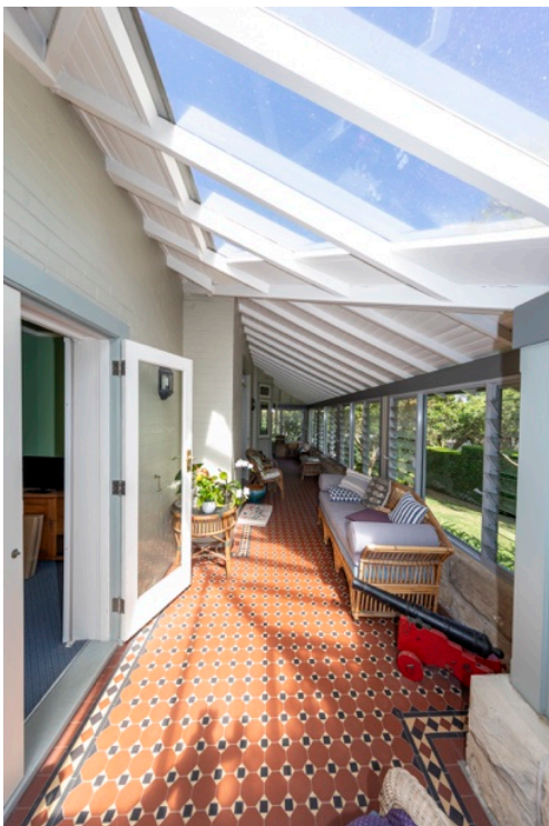
Figure 32: (Left) Enclosed front verandah looking west. Note modern glazed doors at left, and glazed roofing in the foreground.
