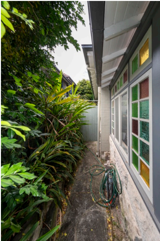
Figure 21: (Left) View of the eastern elevation of the house, with the enclosed front verandah in the foreground
