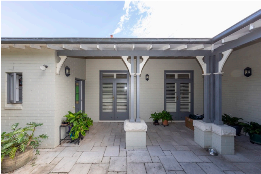
Figure 24: View of the rear elevation. The setback wall is the original rear wall of the house, which was reconstructed during the 1997 alterations and additions.
