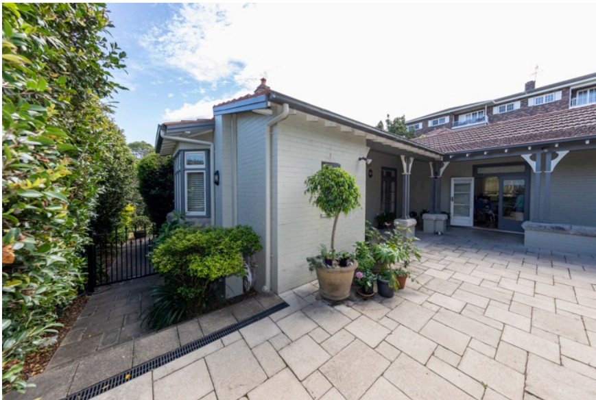
Figure 22: View of the western side elevation (at left) and part of the rear (southern) elevation of the house
