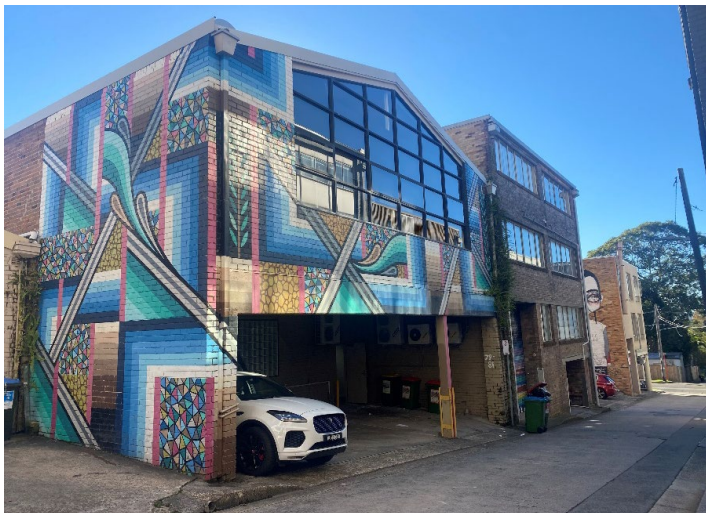
Figure 6 Vehicular access to the site from Atchison Lane Source: Ethos Urban
