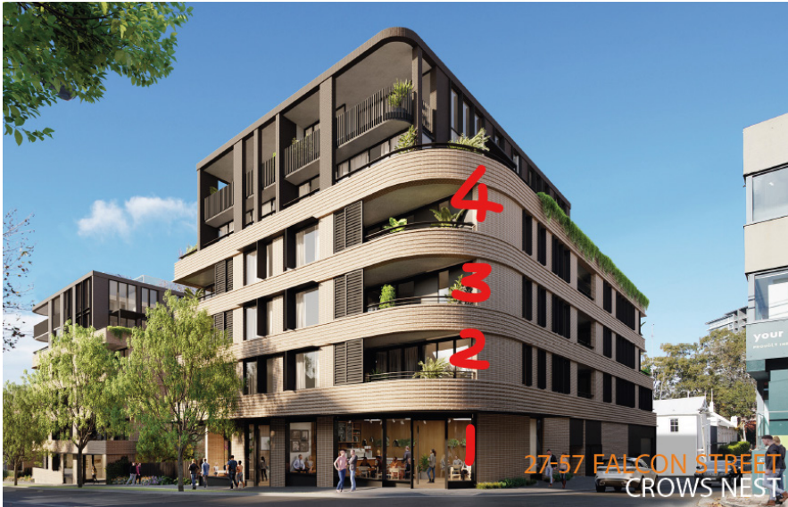
NEIGHBOURING SITE TO THE EAST (NOW UNDER CONSTRUCTION)
