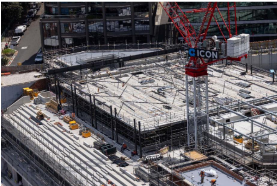
Aerial View – 25m Pool Hall and Grandstands 13/12/23
