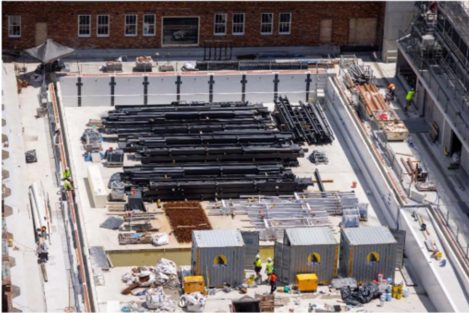
Aerial View – 50m Pool East 13/12/23
