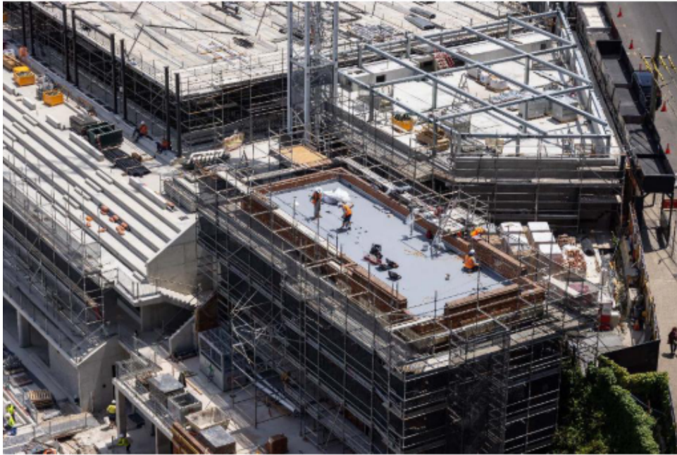
Aerial View – Eastern Stair Tower 13/12/23
