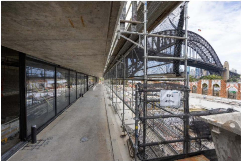
Level 2 Gym Area Glazing 06/11/23
