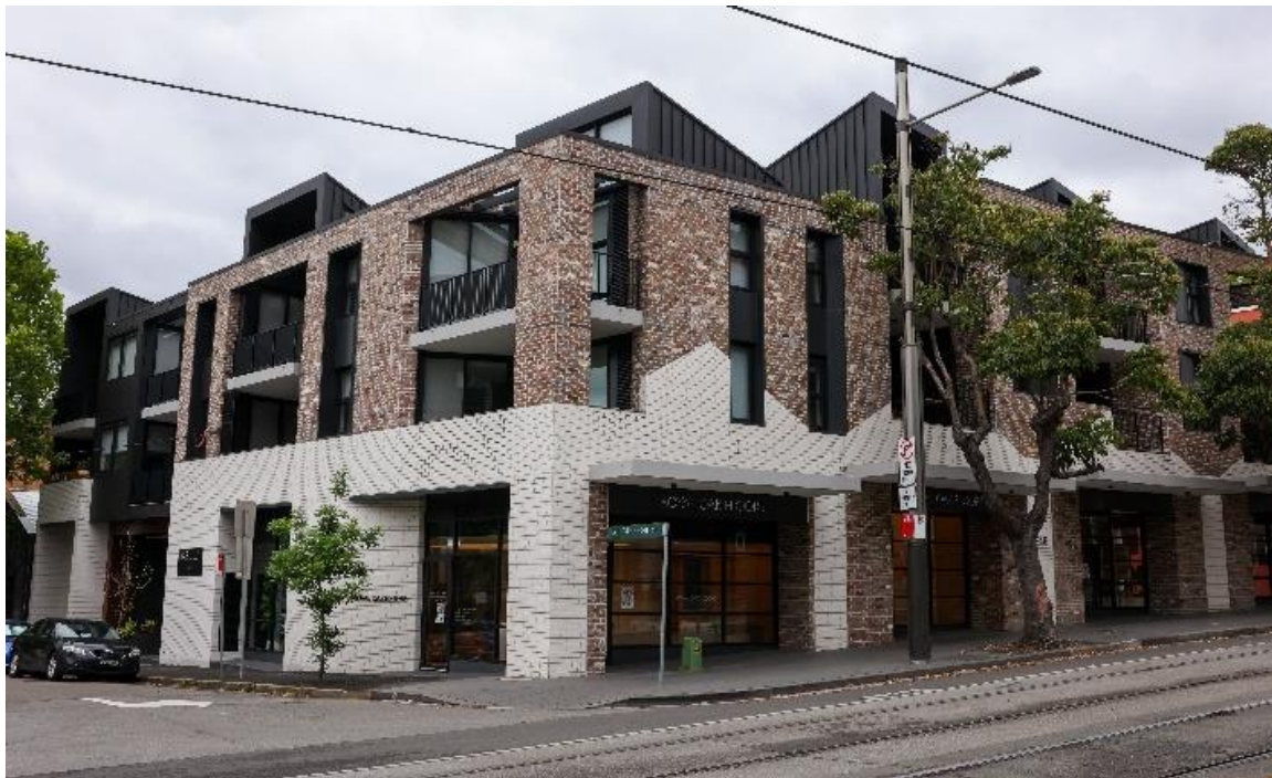
Figure 4: Shop top housing in Surry Hills
