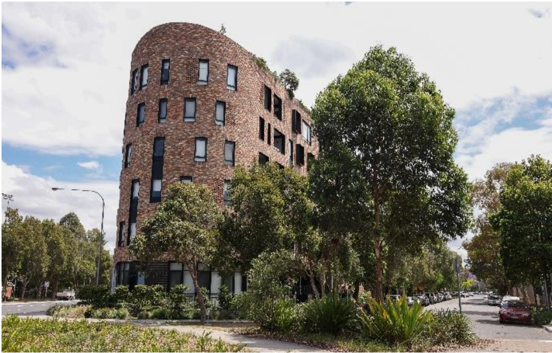
Figure 4: Residential flat building on Huntley Street, Alexandria
