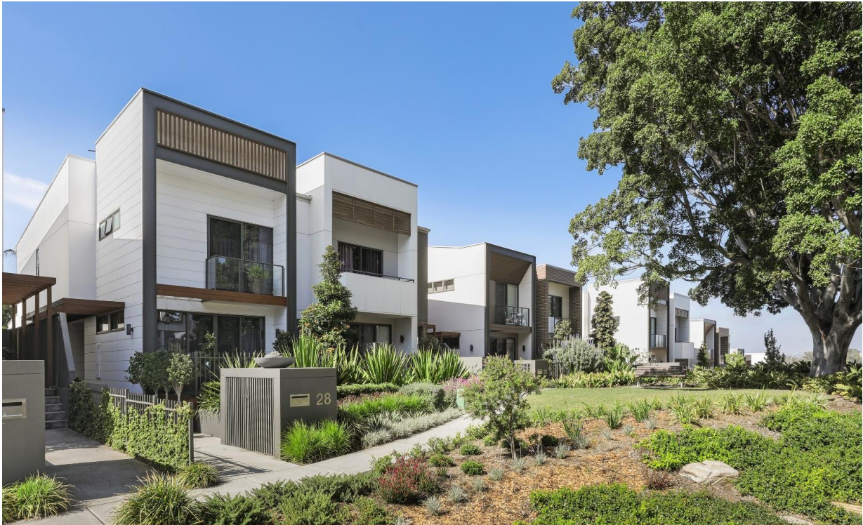
Figure 12: Dual occupancy housing in Ryde
