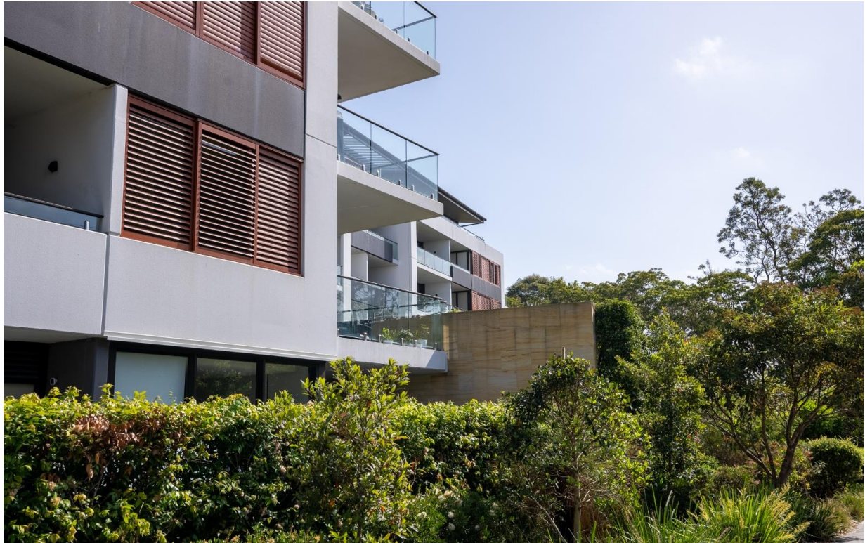
Figure 1: Residential flat building in Lane Cove
