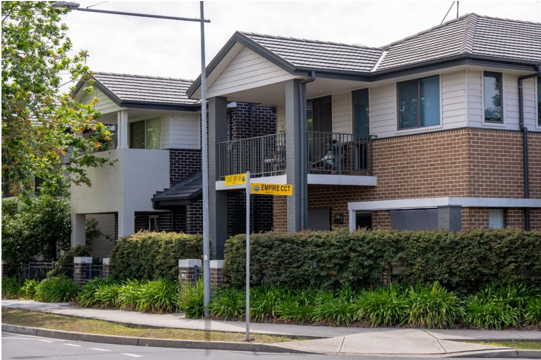
Figure 9: Manor house in Thornton
