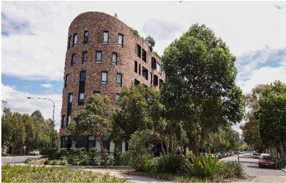
Figure 4: Residential flat building on Huntley Street, Alexandria
