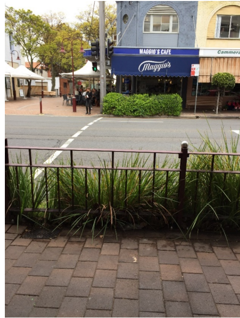
Figure 20 Protection barriers The design of protection barriers for pedestrians on busy Miller Street, Cammeray successfully integrates high quality design and safety.
