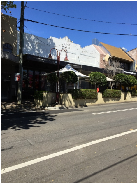
Figure 16 Building stock character There is good character building stock which has an appealing human scale and contributes to the Crows Nest Town Centre atmosphere
