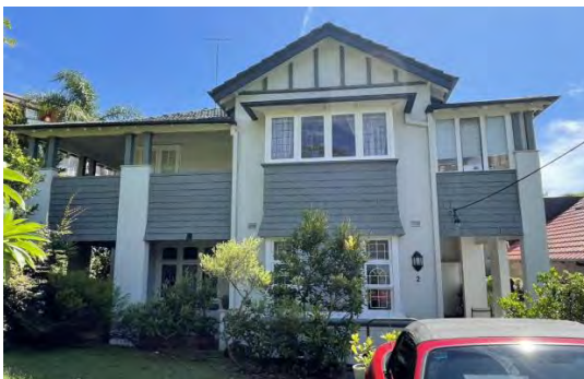
Figure 5.44 View of the primary elevation of 125 Holt Avenue, looking north.
