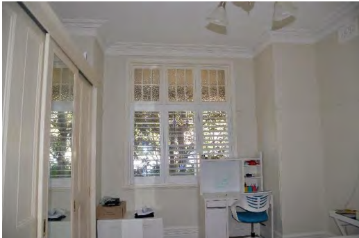
Figure 5.21 View of the timber casement windows to the front bedroom.
