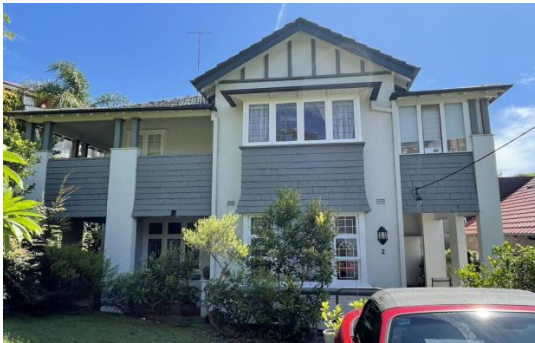
Figure 5.23 View of the primary elevation of 125 Holt Avenue, looking north.
