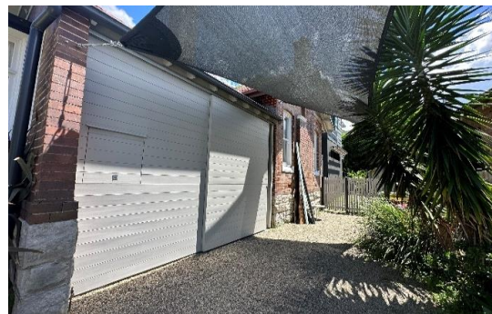
Figure 5.14 East elevation with contemporary sliding doors.
