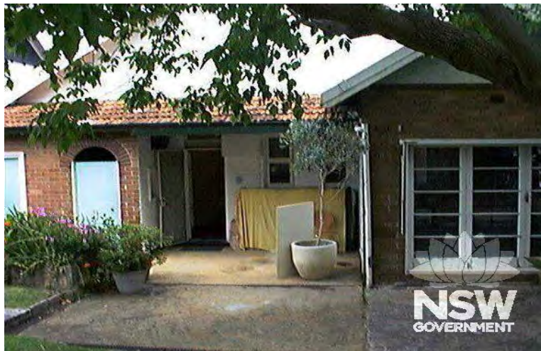
Figure 6.3 Detail of 23 Bannerman Street. (Source: NSW State Heritage Inventory)
