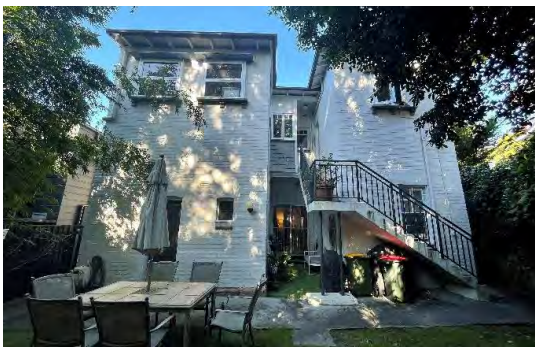
Figure 5.46 View of the rear elevation, facing south-west.
