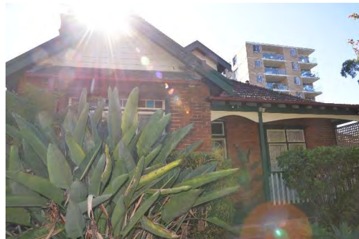
Figure 5.4 View of the western elevation of the dwelling.
