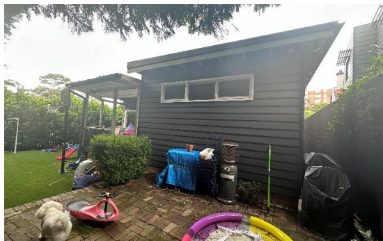
Figure 5.12 Rear (northern) elevation.
