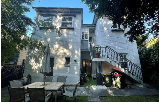
Figure 5.25 View of the rear elevation, facing south-west.
