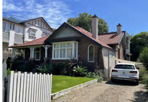
Figure 5.43 View showing the eastern elevation, roof form and temporary car shade, looking northwest.
