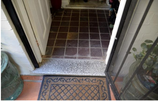
Figure 5.31 First floor apartment to west— terrazzo threshold.
