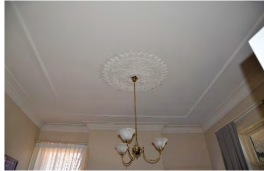
Figure 5.26 View of original plaster ceiling rose to the front section.
