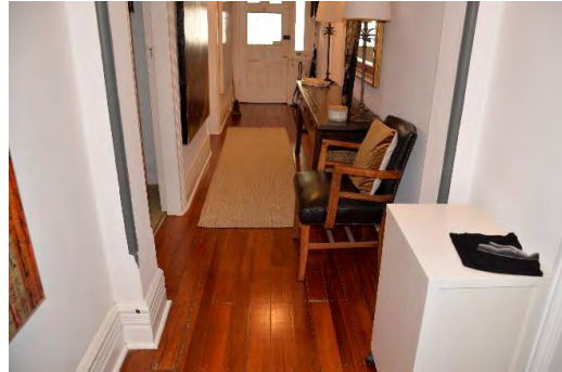
Figure 5.14 View of the original timber floorboards.
