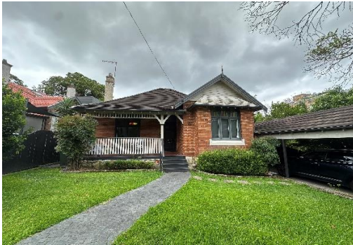
Figure 5.1 View of the primary elevation of 121 Holt Avenue, looking north.
