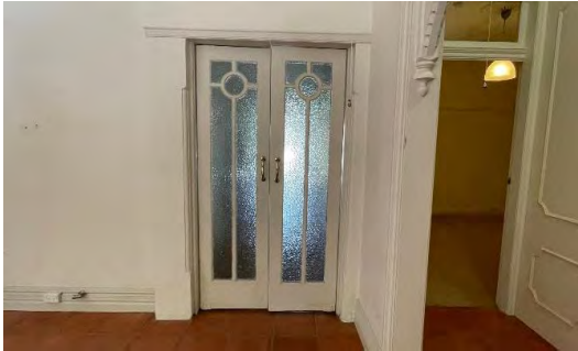
Figure 5.37 View to an internal door with stop chamfering detailing along the doorway.
