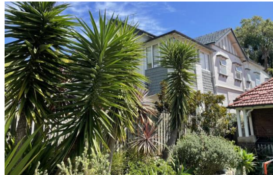
Figure 5.24 View showing a detail of the upper storey of the eastern elevation. The enclosed balcony, with timber detailing, is visible.
