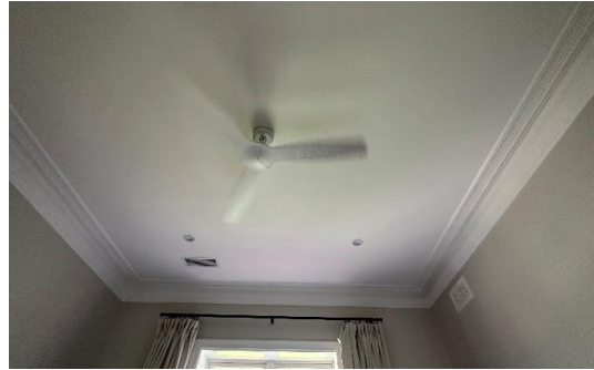
Figure 5.20 New ceilings in the front bedroom.
