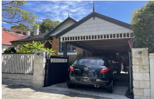
Figure 5.2 View showing the carport with matching timber shingles, looking northwest.
