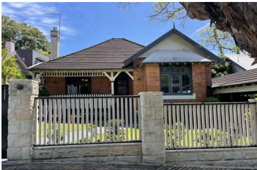
Figure 5.39 View of the primary elevation of 121 Holt Avenue, looking north.
