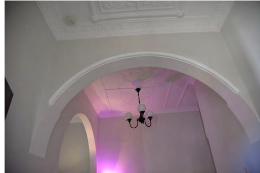
Figure 5.49 Ground floor apartment to east—arched entryway with stop chamfer detailing.
