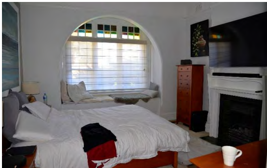
Figure 5.9 View of the original bay windows and arch with stop chamfer detailing to the front bedroom.
