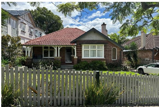
Figure 5.13 View of the primary elevation of 123 Holt Avenue, looking north.
