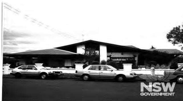
Figure 6.1 Primary façade of 7 Cranbrook Avenue, 'Belvedere'. (Source: NSW State Heritage Inventory)
