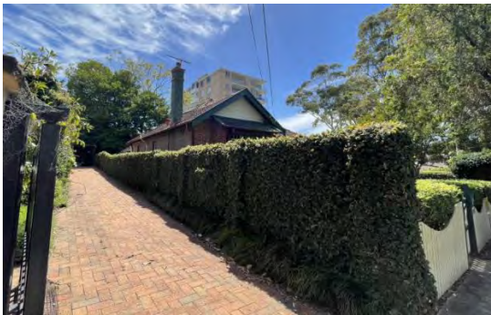
Figure 5.3 View of the western elevation and the original chimney, looking northeast.
