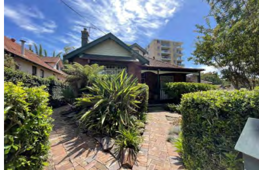
Figure 5.2 View showing the verandah and access path.
