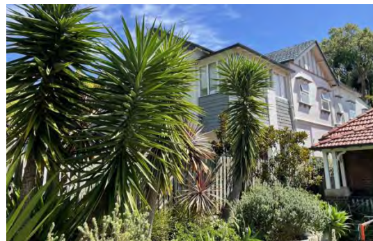
Figure 5.45 View showing a detail of the upper storey of the eastern elevation. The enclosed balcony, with timber detailing, is visible.
