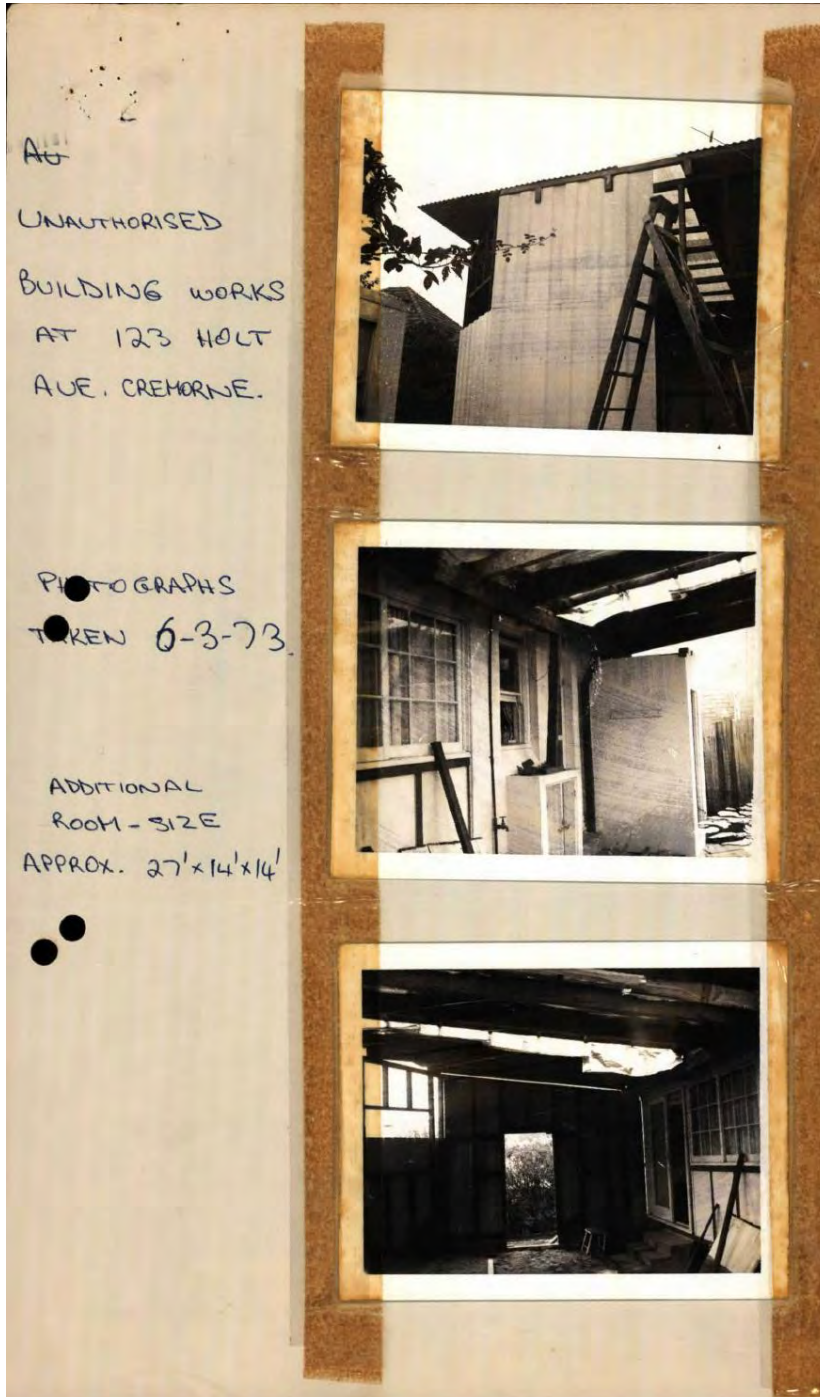
Figure 4.25 Three views showing unauthorised building works, 123 Holt Avenue, 6 March 1973. (Source: North Sydney Council, P339/123/3)
