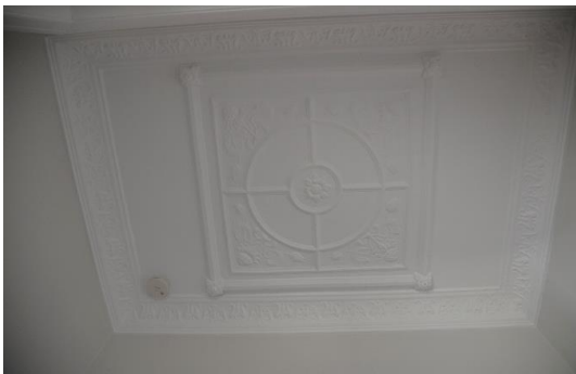
Figure 5.27 Ground floor apartment to east—original decorative plaster ceilings.
