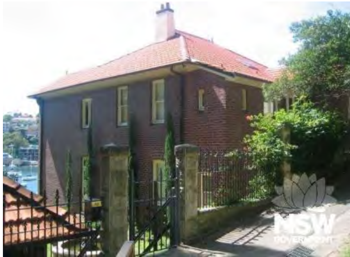
Figure 6.9 'Balangowan', Bromley Avenue. (Source: NSW State Heritage Inventory)
