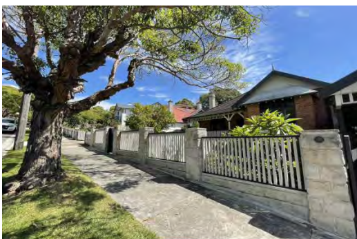
Figure 5.41 View showing the property from the street, with stone fence and timber balustrade, looking northwest.
