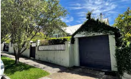
Figure 5.31 View showing the garage addition, looking northwest.
