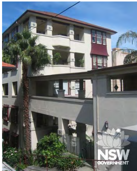
Figure 6.14 ‘Mayfair Flat Building’, 86 Milson Road, Cremorne Point. (Source: NSW State Heritage Inventory)
