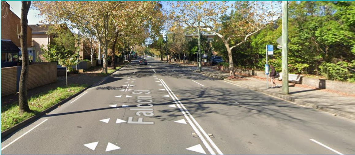
Figure 2-7 Falcon Street, viewed westwards towards West Street (Image Source: Google Street View)
