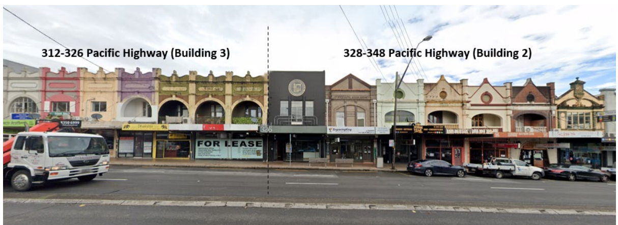
Figure B2.4: Heritage façade along Pacific Highway at Crows Nest
