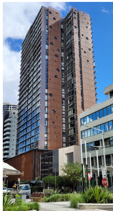
Picture 6 Quest apartments (looking northwest)
