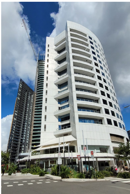
Picture 5 Existing building (looking southwest)
