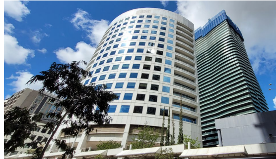
Picture 2 Existing building (looking south-east)
