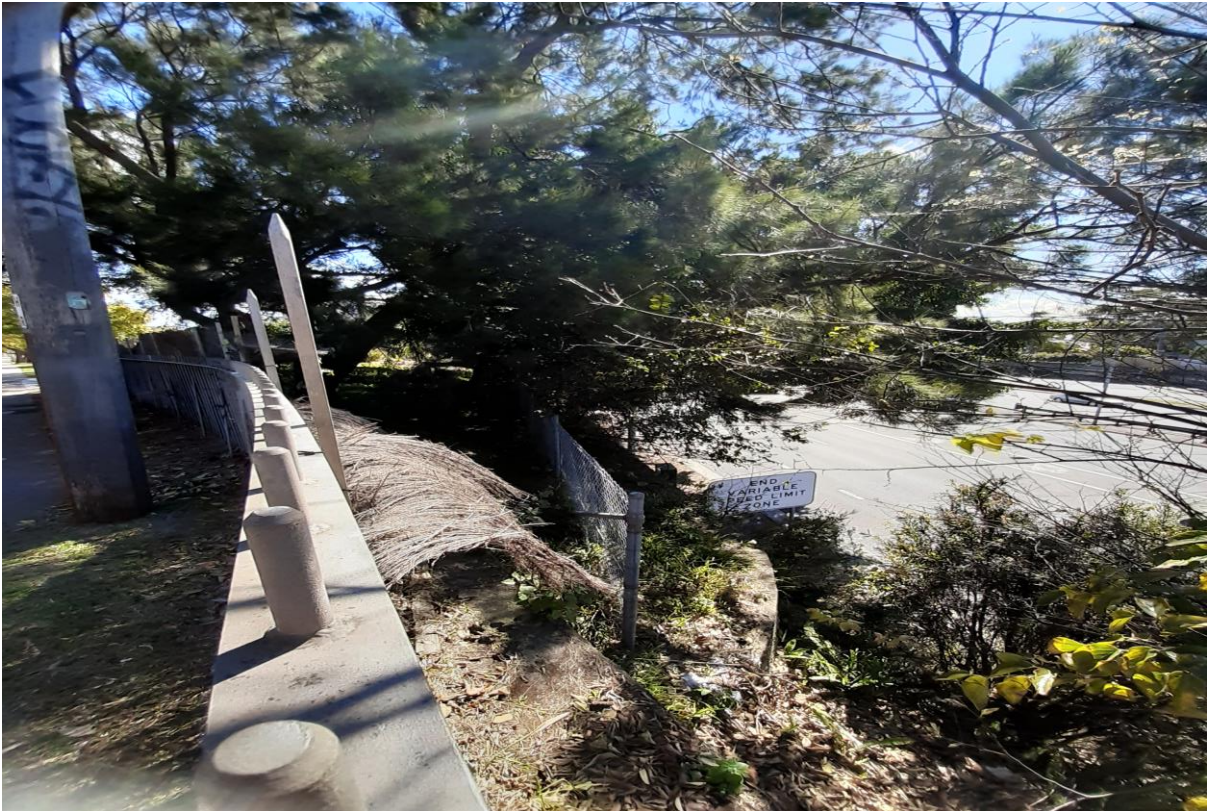
Photo 5 – Proposed Location of RMS noise wall at North Eastern end of Chandos Street adjacent to Warringah Freeway
