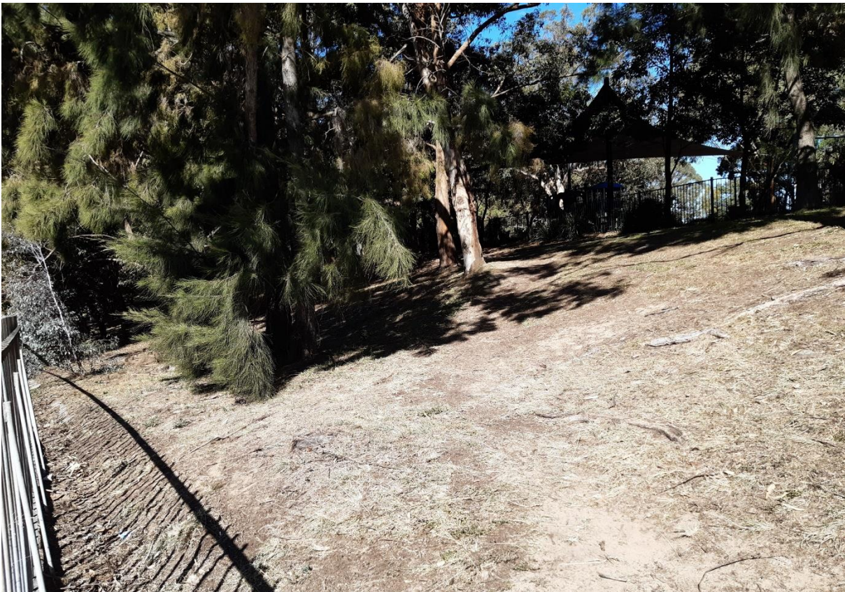
Photo 7 – Proposed Location of RMS noise wall at North Eastern end of St Thomas Rest Park adjacent to Warringah Freeway
