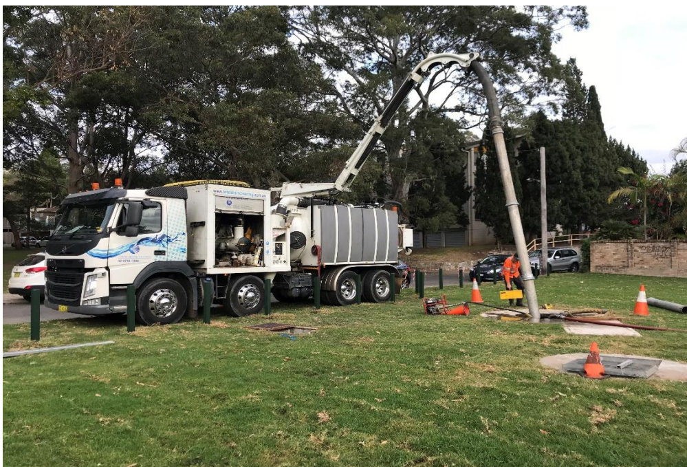
GPT being cleaned (Little Young Street 2018)
