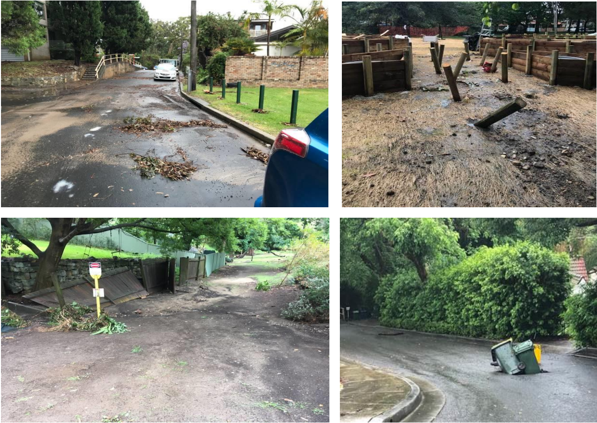
Flooding Damage examples in North Sydney LGA – 27 November 2018 – 1:100 year storm event Figure 1. Map showing Inlets in each Risk Category below.
