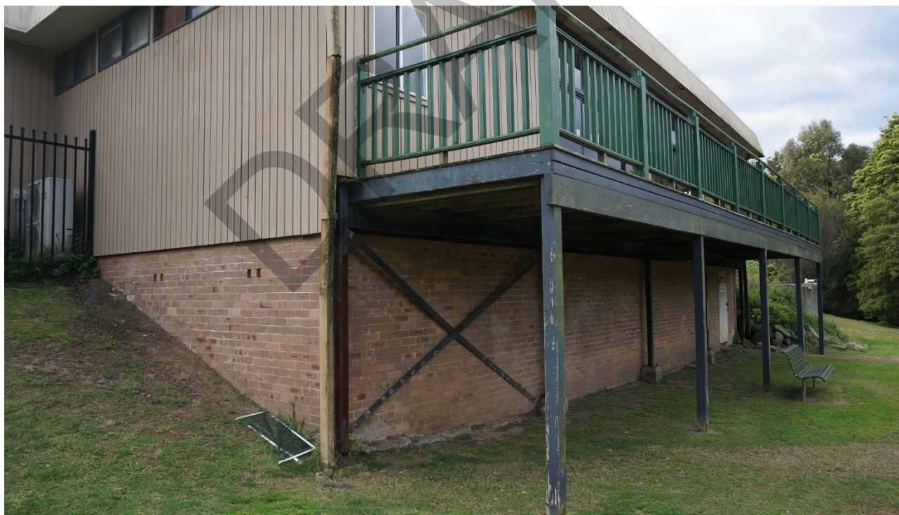
10. View of the rear of the club house building showing the bricked-in sub-floor area.
