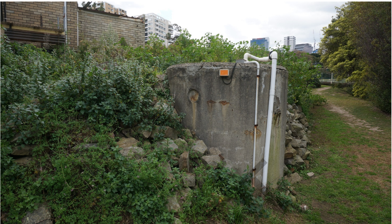
15. Septic tank located at the south east corner of the building. A second septic tank is present is located in this area but is not visible in this photograph.
