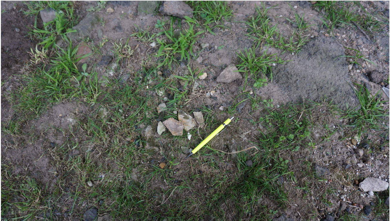
13. Fragments of suspected asbestos cement sheet on the ground surface on the southern side of the building (pen for scale).
