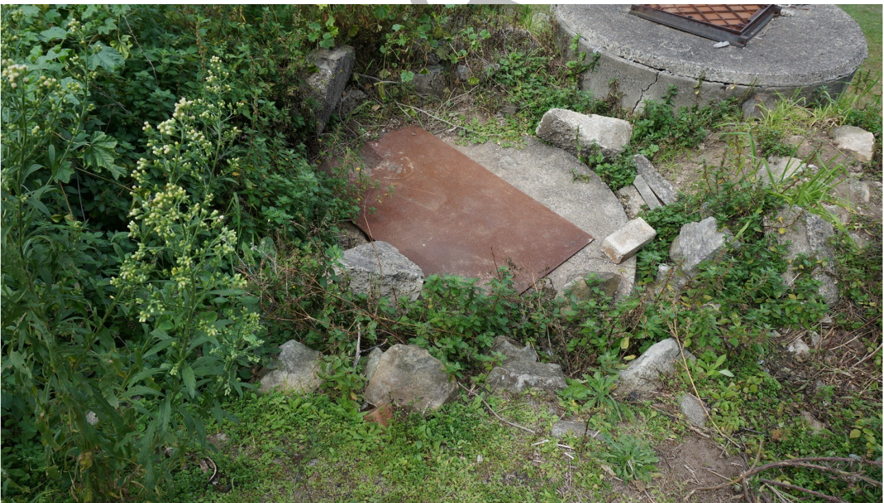
16. View from above of two septic tanks at the south east corner of the building.
