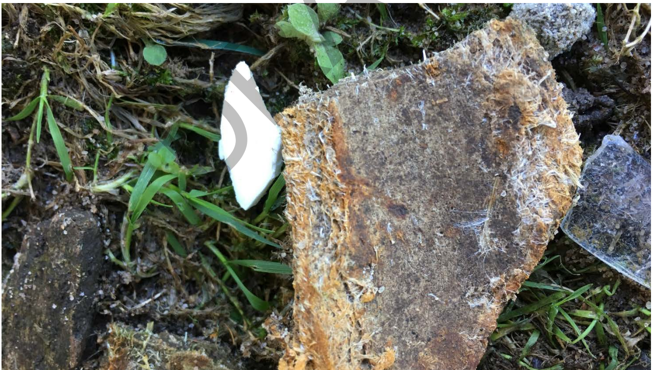
14. Close up of suspected asbestos cement sheet fragment. Laboratory analysis confirmed the presence of chrysotile asbestos in the cement sheet.
