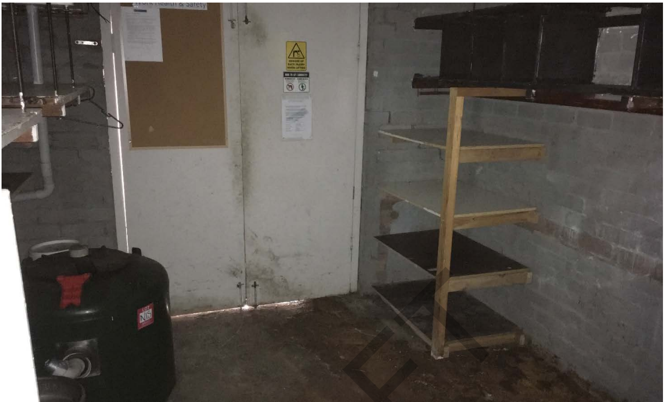
19. View of interior of storeroom accessed from inside the building. The area housed wastewater treatment equipment.
