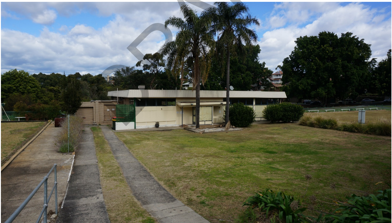
8. View to south from Woolcott Street to the club house building. Two storage areas were present on the eastern side of the building, and one storage area was present on the western side of the building (not visible in this photograph).
