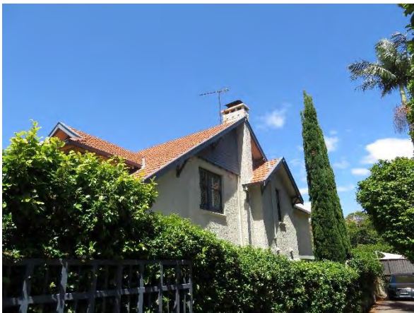
Figure 3.7 Detail view of the northern elevation of 6 Hayes Street. Note the prominent cypress trees, gable detail, chimney and roughcast exterior render. (Source: GML, 2018)
