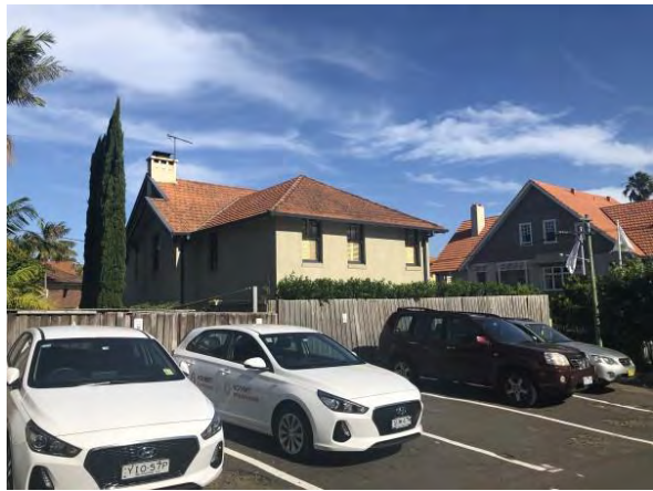
Figure 4.22 View of 6 Hayes Street showing the north and west elevations, taken from a neighbouring property. (Source: GML, 2018)
