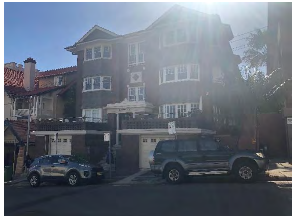
Figure 5.9 Kcot Sedar, 4 Hayes Street. (Source: GML, 2018)
