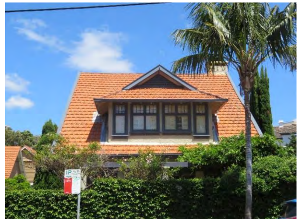
Figure 4.16 6 Hayes Street, detail of east elevation. (Source: GML, 2018)
