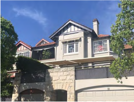
Figure 4.9 Example of a building on Wallaringa Avenue. (Source: GML, 2018)
