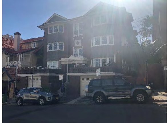
Figure 4.7 Kcot Sedar, 4 Hayes Street (Source: GML, 2018)
