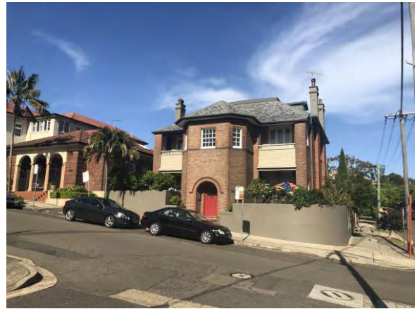
Figure 4.6 Corner of Hayes Street and Lower Wycombe Road. The former post office is on the left. (Source: GML, 2018)
