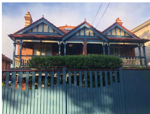
Figure 5.17 51 and 53 Kurraba Road. (Source: GML, 2019)
