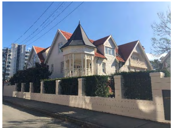
Figure 4.9 Wallaringa Mansions 1 Wallaringa Avenue. (Source: GML, 2018)
