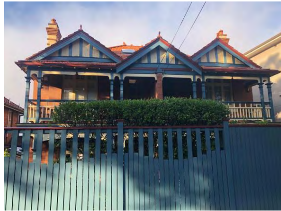
51 and 53 Kurraba Road showing decorated gable ends. (Source: GML, 2019)
