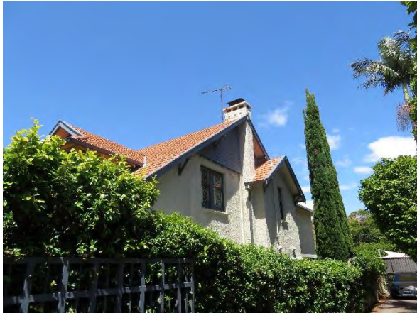
Figure 4.19 Detail view of the northern elevation of 6 Hayes Street. Note the prominent cypress trees, gable detail, chimney and roughcast exterior render. (Source: GML, 2018)
