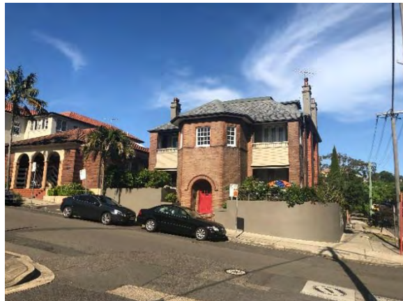
Figure 4.13 17 Hayes Street (Source: GML, 2018)
