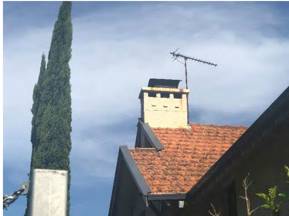
Figure 4.20 Detail view of the chimney at 6 Hayes Street. (Source: GML, 2018)
