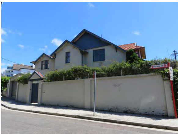
Figure 4.17 6 Hayes Street, south elevation viewed from Manns Avenue. (Source: GML, 2018)
