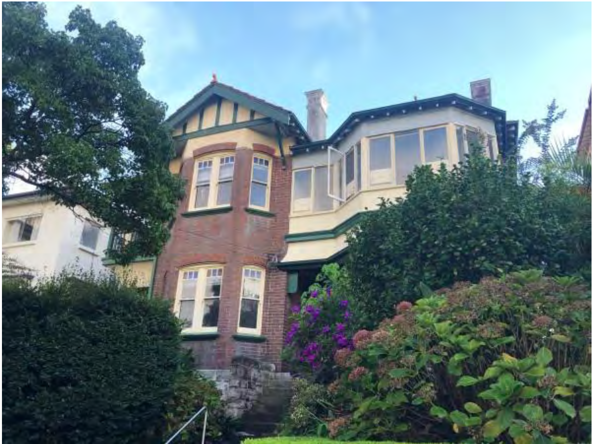
18 Lower Wycombe Road as viewed from the street. (Source: GML, 2019)
