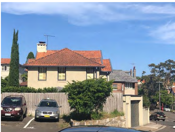
Figure 3.9 View of the rear of 6 Hayes Street, from the neighbouring property at 2 Manns Avenue. (Source: GML, 2018)
