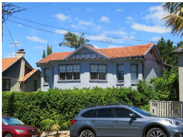
Figure 3.10 Exterior view of 8 Hayes Street. (Source: GML, 2018)
