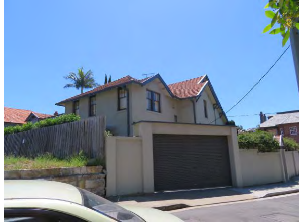
Figure 3.6 Rear of 6 Hayes Street from Manns Avenue, showing driveway entry. (Source: GML, 2018)
