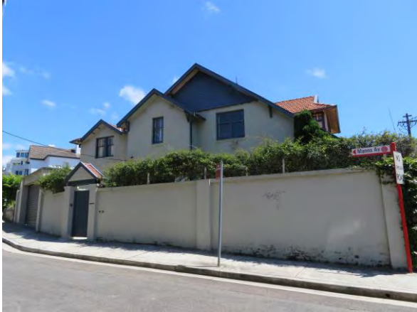
Figure 3.5 6 Hayes Street, south elevation viewed from Manns Avenue. (Source: GML, 2018)
