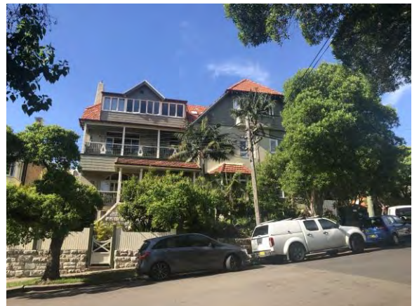
View of the building from Lower Wycombe Road. (Source: GML, 2018)
