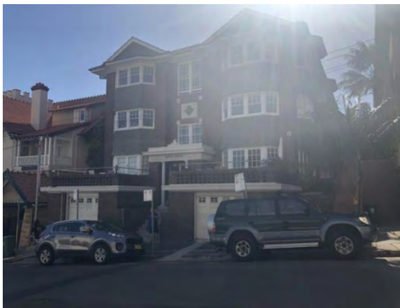
Kcot-Sedar viewed from Hayes Street. (Source: GML, 2018)
