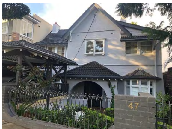
Figure 5.16 47 Kurraba Road. (Source: GML, 2019)
