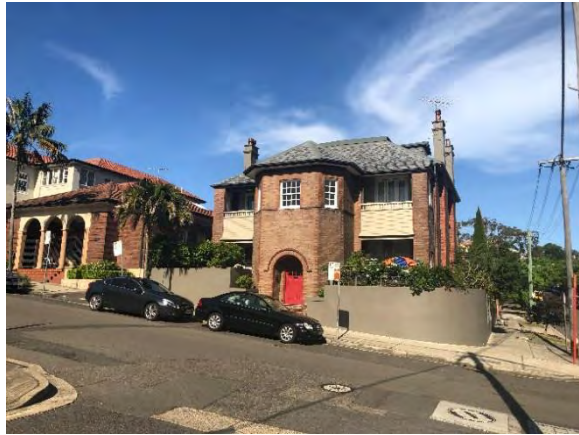
Figure 5.23 17 Hayes Street. (Source: GML, 2018)
