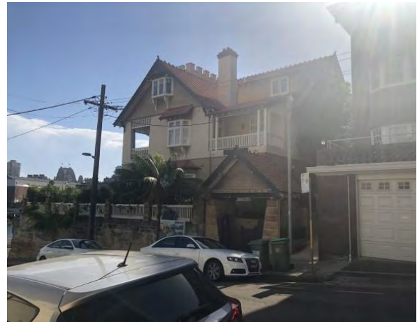
The Hastings viewed from Hayes Street. (Source: GML, 2018)
