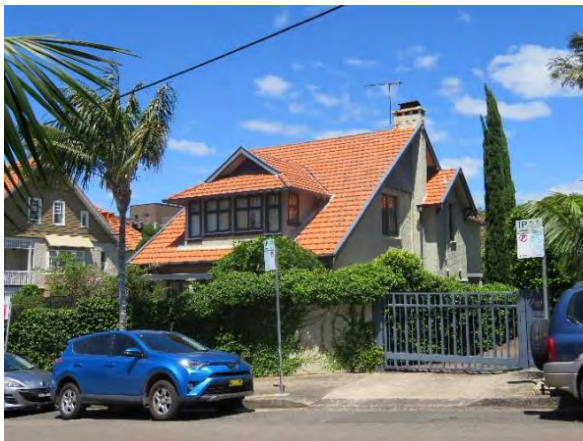
Figure 4.15 6 Hayes Street, east elevation from across Hayes Street. (Source: GML, 2018)
