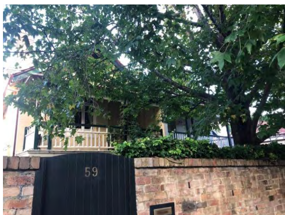
Figure 5.20 59 Kurraba Road. (Source: GML, 2019)
