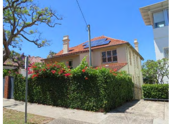
Figure 4.19 11 Lower Wycombe Road (contributory). (Source: GML, 2018)
