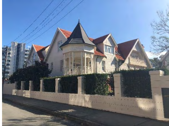
Figure 5.11 Wallaringa Mansions from Wallaringa Avenue. (Source: GML, 2018)
