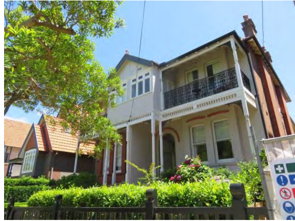
Figure 4.10 Example of a building on Lower Wycombe Road. (Source: GML, 2018)
