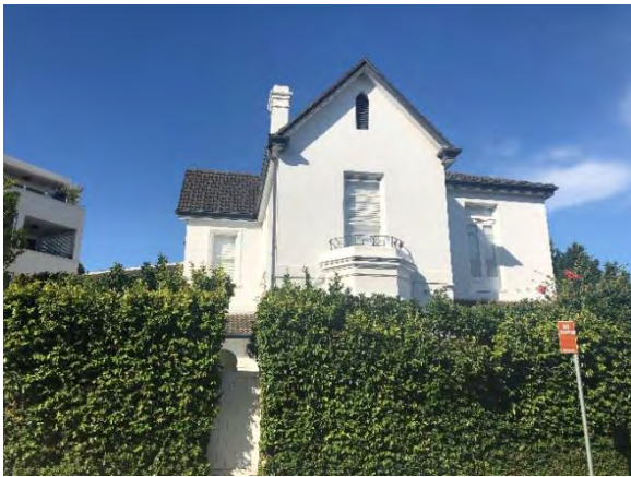
Figure 5.24 2 Manns Avenue. (Source: GML, 2018)
