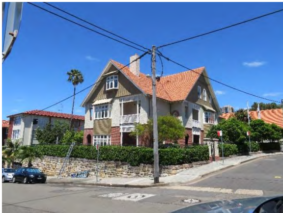
Figure 5.8 11 Manns Avenue (corner of Hayes Street and Manns Avenue). (Source: GML, 2018)
