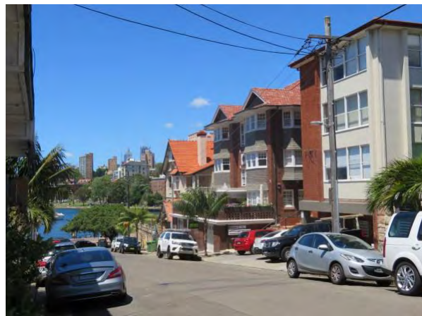
View of Kcot-Sedar further up Hayes Street showing the frontage. (Source: GML, 2018)
