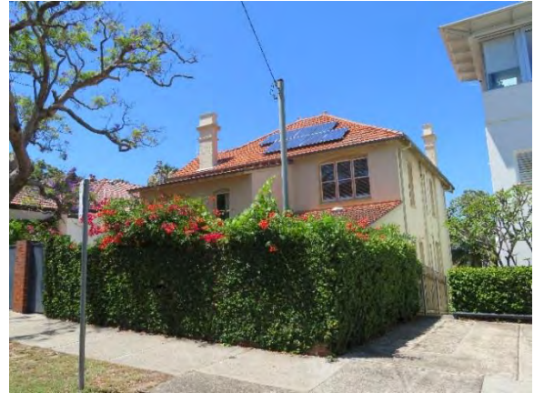
Figure 5.29 11 Lower Wycombe Road (contributory). (Source: GML, 2018)
