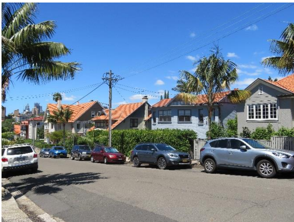
Figure 3.1 View of the subject properties within their immediate context, looking south down Hayes Street. No. 8 is in the centre with No. 6 just beyond. (Source: GML, 2018)
