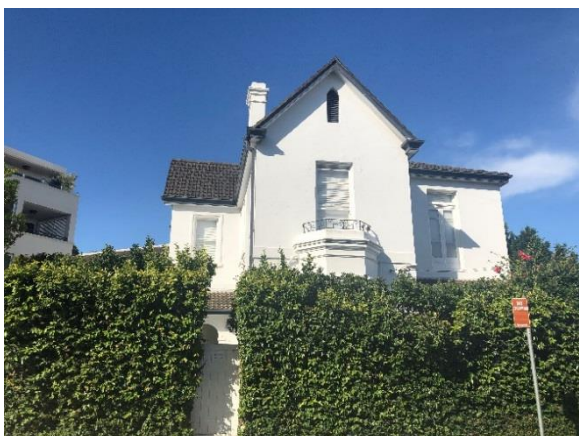
Figure 4.14 2 Manns Avenue. (Source: GML, 2018)
