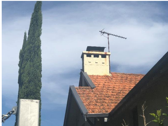
Figure 3.8 Detail view of the chimney at 6 Hayes Street. (Source: GML, 2018)
