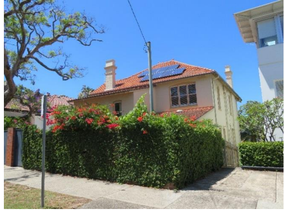
Figure 4.19 11 Lower Wycombe Road (contributory). (Source: GML, 2018)
