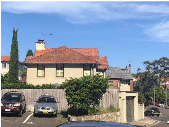
Figure 3.9 View of the rear of 6 Hayes Street, from the neighbouring property at 2 Manns Avenue. (Source: GML, 2018)
