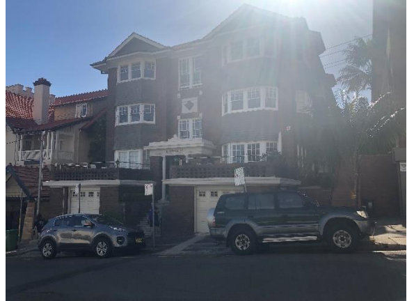
Figure 4.7 Kcot Sedar, 4 Hayes Street (Source: GML, 2018)
