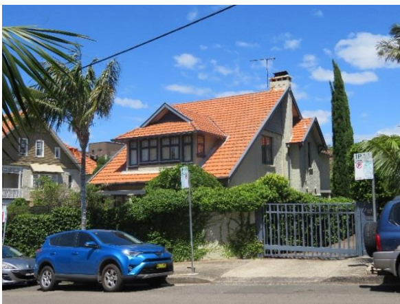
Figure 3.3 8 Hayes Street. (Source: GML, 2018)
