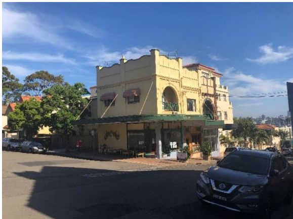
Figure 4.12 11 - 15 Hayes Street. (Source: GML, 2018)
