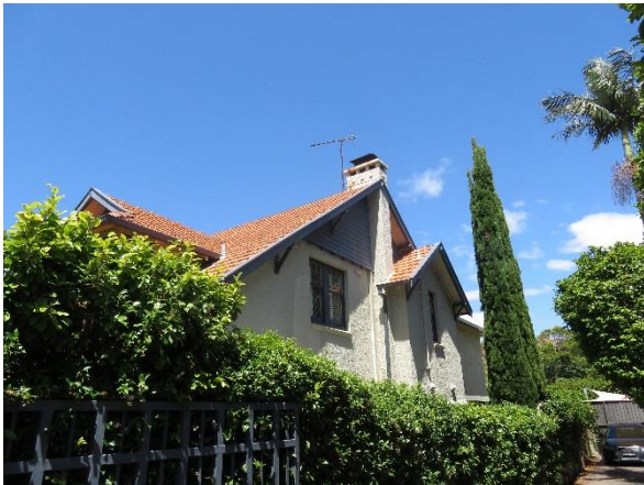
Figure 3.7 Detail view of the northern elevation of 6 Hayes Street. Note the prominent cypress trees, gable detail, chimney and roughcast exterior render. (Source: GML, 2018)
