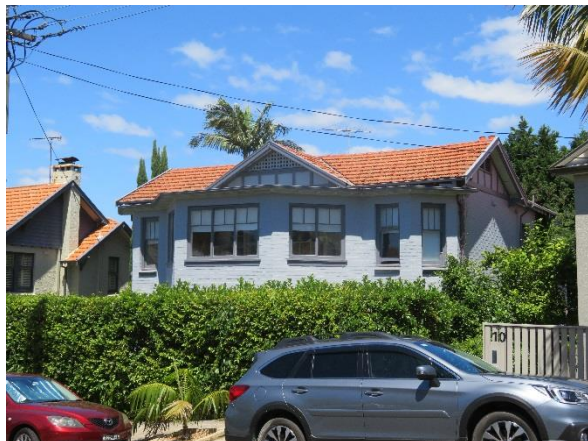
Figure 3.10 Exterior view of 8 Hayes Street. (Source: GML, 2018)
