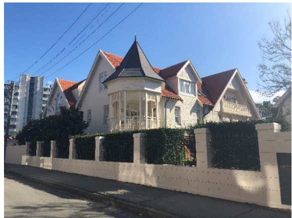
Figure 4.9 Wallaringa Mansions 1 Wallaringa Avenue. (Source: GML, 2018)
