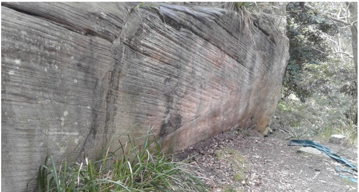
Before and after photos of typical instance of Graffiti in North Sydney in Bushland – Rock face at Primrose Park, Cremorne.
