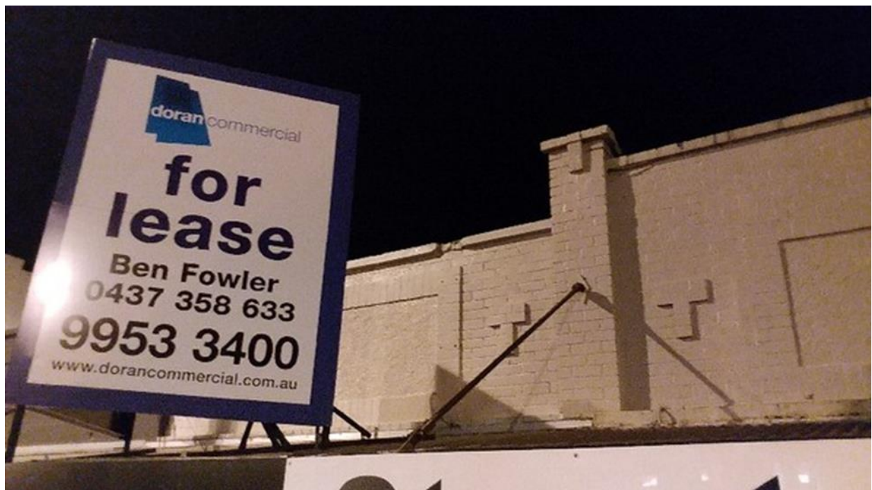
Before and after photos of typical instance of Graffiti in North Sydney on Private Property in difficult to access places. Council needs Property owners consent to access and remove graffiti in these types of instances - instances (shop on 236 Military Road, Neutral Bay).
