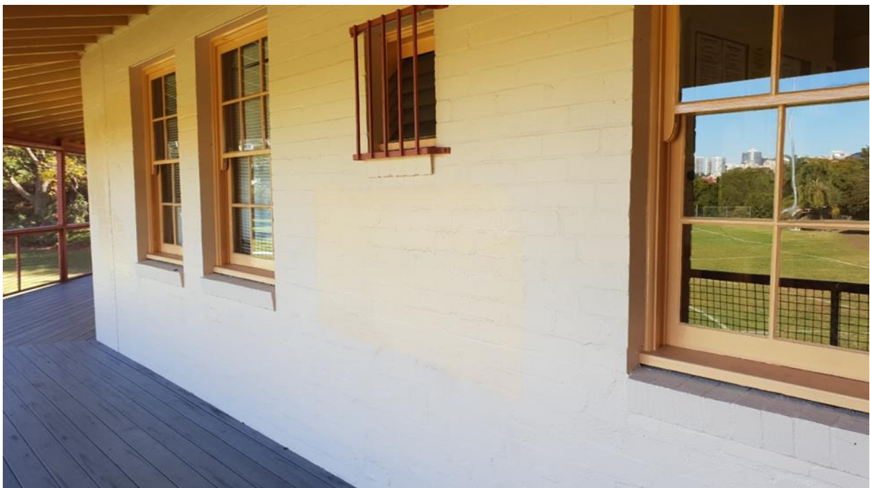
Before and after photos of typical instance of Graffiti in North Sydney on Council Facilities – Forsyth Park Community Centre, Neutral Bay.
