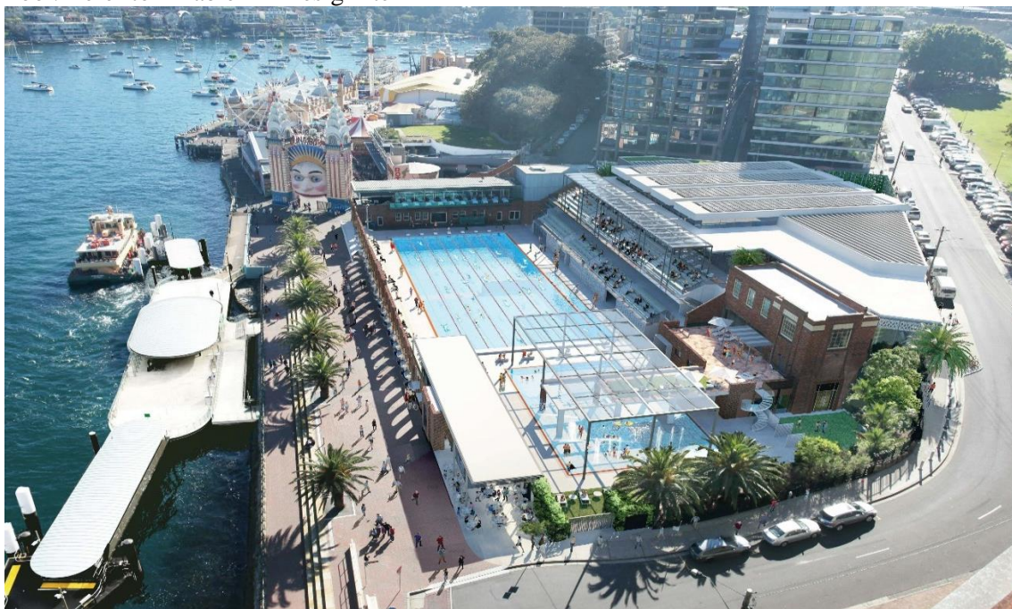
Figure 2. Aerial View looking at the Eastern Sundeck and Shade canopy over the Children's Swimming Pool. Refer to – Table 1 – Design Item 2
