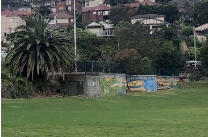
① view looking east onto water tanks
