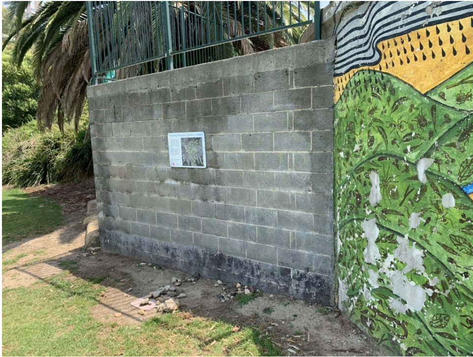
Photograph 3: Pump room a western end of tanks
