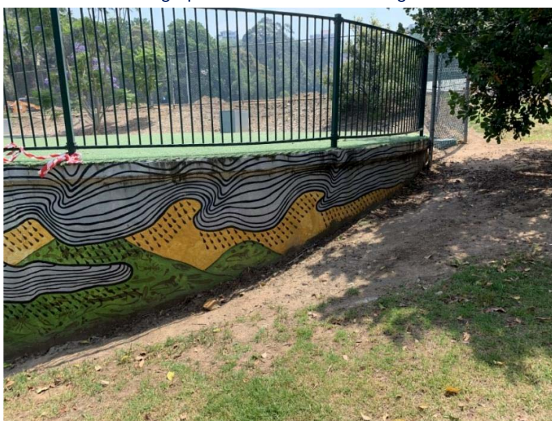
Photograph 2: Tanks recessed into embankment
