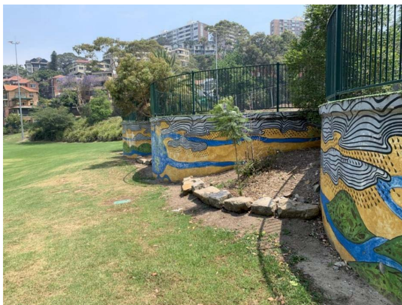
Photograph 1: View of tanks looking west
