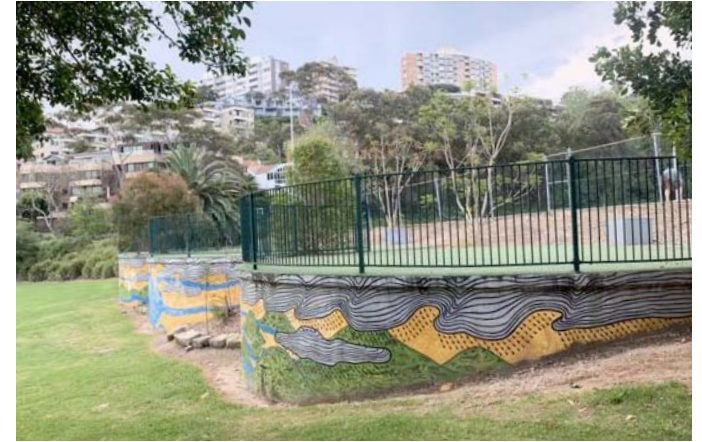
③ view looking west onto water tanks
