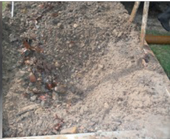
Litter Basket full of silt prior to cleaning
