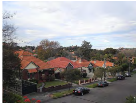
Figure B-13.13: Buildings from the nineteenth and early twentieth centuries often have steep pitches and formal geometry that combines to give a distinctive skyline.
