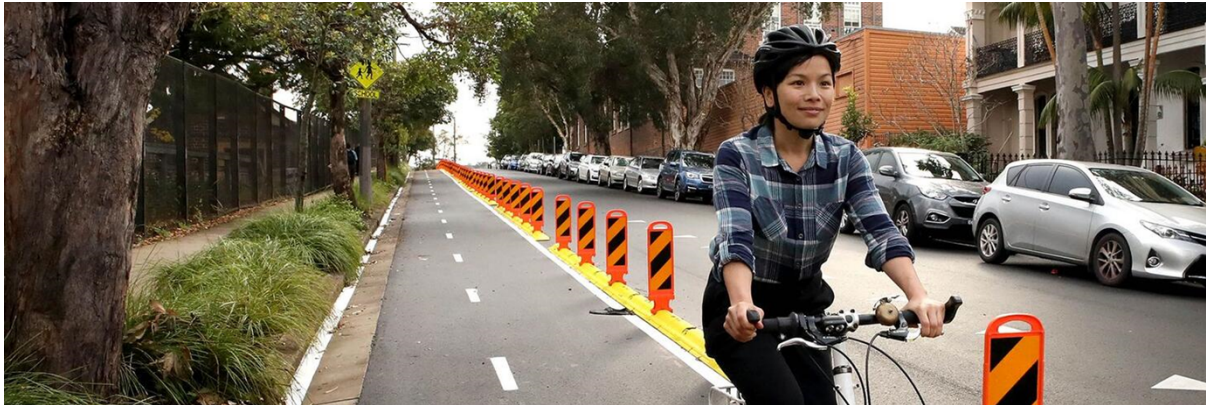
Image 10. Temporary on road separated cycleway treatments in City of Sydney LGA
