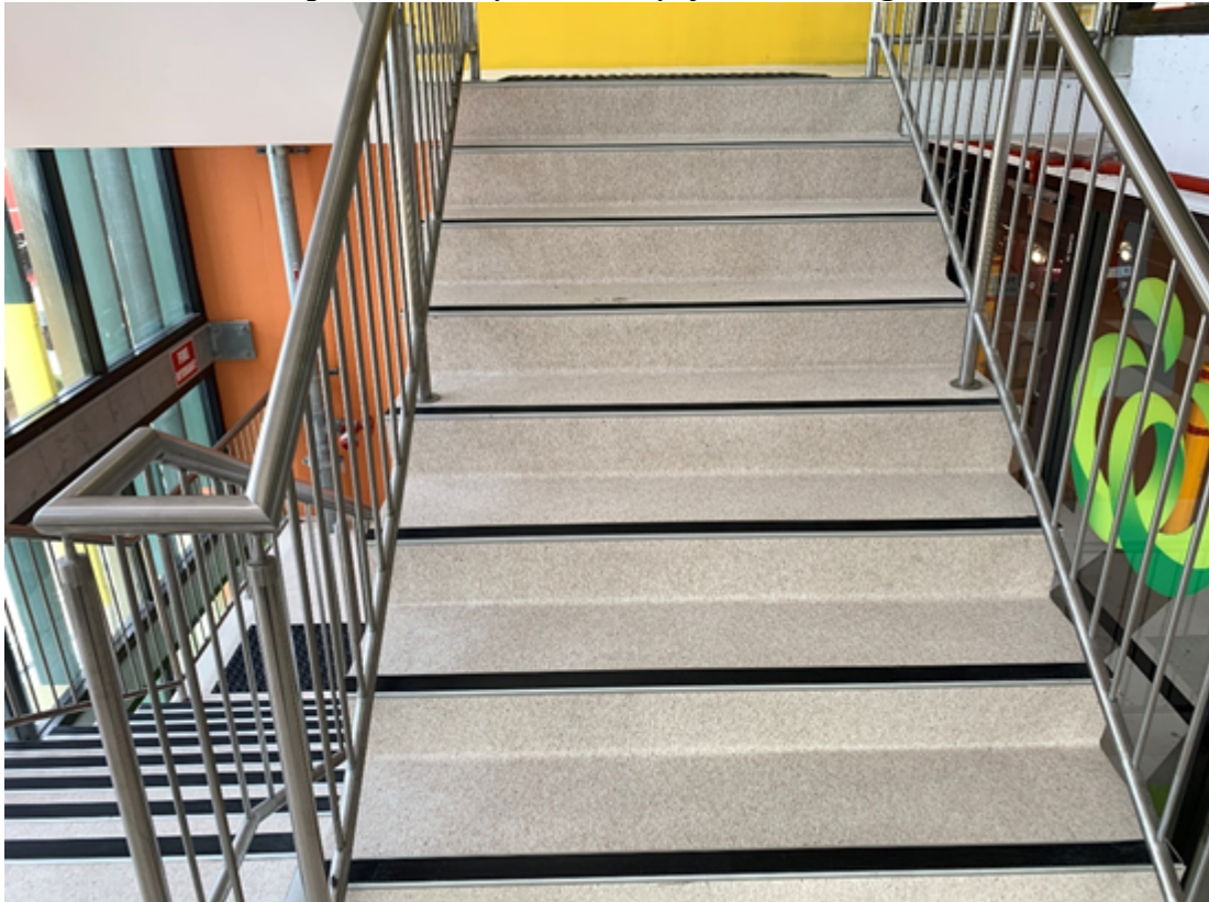
Alexander Street Carpark Stairway – new vinyl floor coverings
