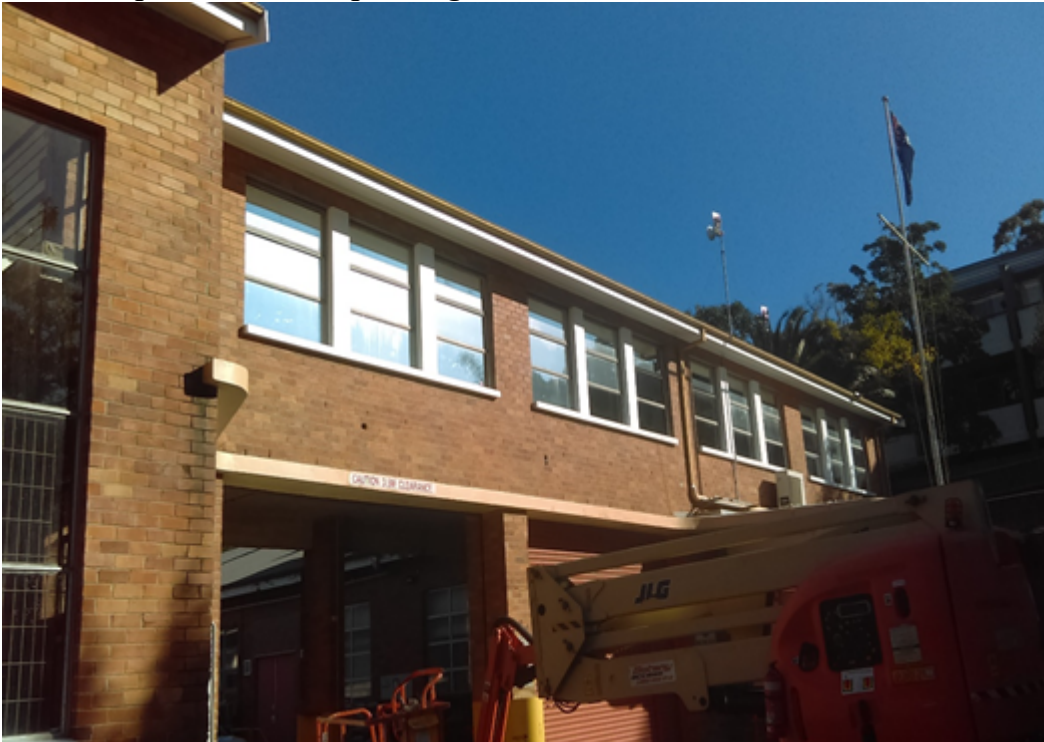
Central Depot – external repainting
