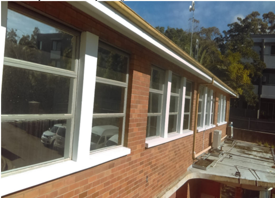
Central Depot – external repainting
