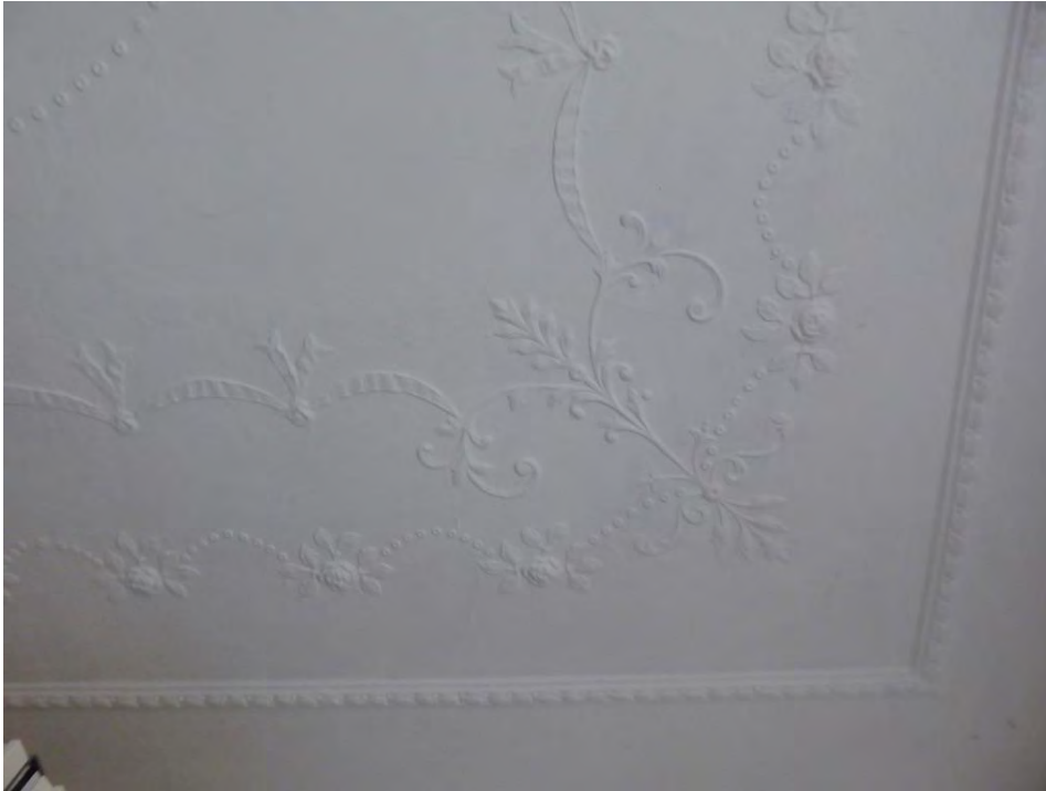
Upper floor bedroom ceiling detail, using moulded fibrous plaster
