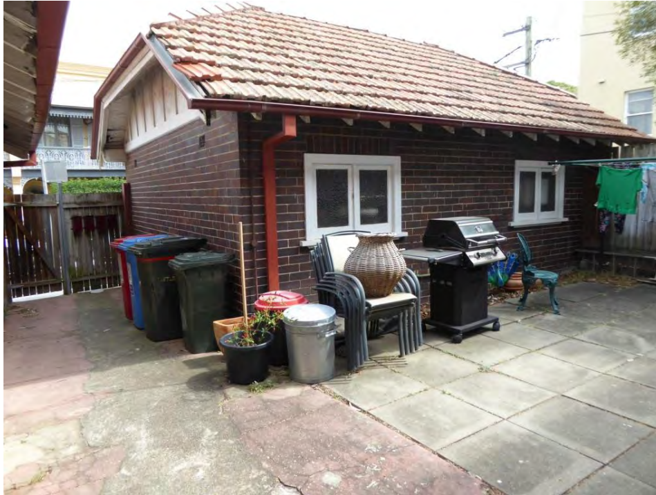
Rear of double garage, with fence to Middle Street at left, and concrete paving
