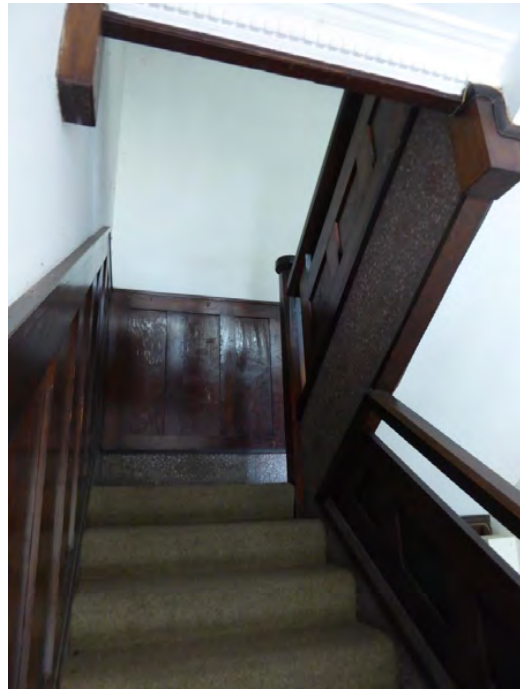
View up lower flight of main stair, balustrade and wainscot
