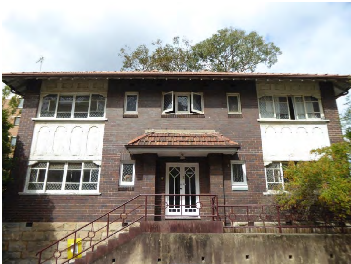
No. 3 Parker Street McMahons Point : principal elevation to Parker Street
