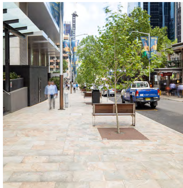
(Left and above) “Bruce” Rock (Austral granite) pavers have been specified throughout the CBD to create a unifying design element within the public domain that is hard wearing and serviceable and therefore suitable for heavy pedestrian traffic.
