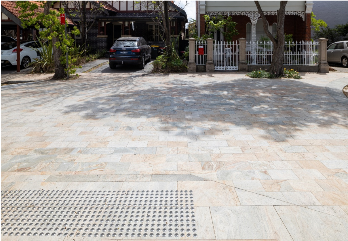
Mount Street at Edward Street – Pedestrian Safety Upgrades (LATM Zone 3 – T.82)- Continuous Footpath treatments and expanded pedestrian crossing areas.
