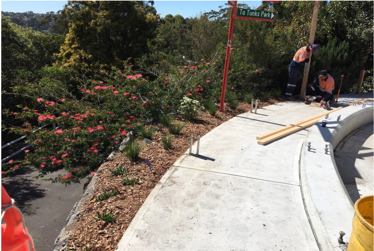
Rowlison Parade – footpath construction
