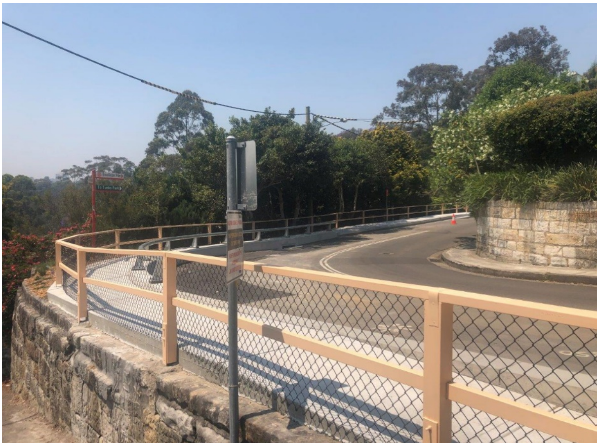
Rowlison Parade – footpath construction
