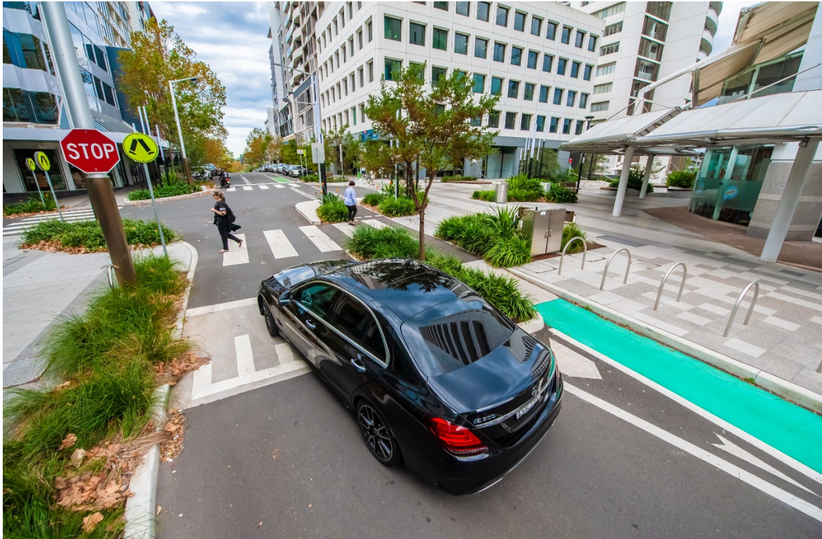
Atchison Street – new Traffic Calming and Pedestrian Crossings / Intersection Upgrade (LATM Zone 2)
