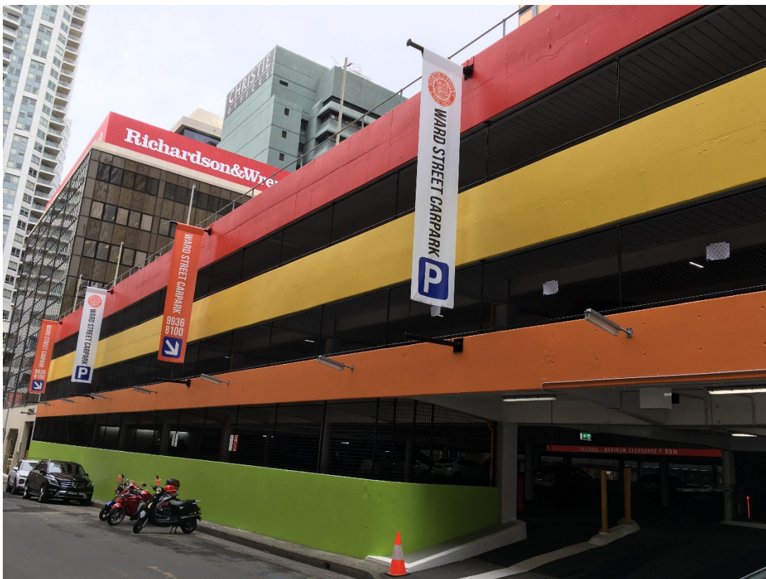
Ward Street Car Park external repainting
