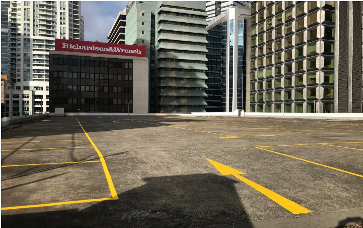
Photo of Ward Street carpark – Roof top level – now used for “Early Bird Parking” new line marking undertaken by Wilson parking as part of the handover to Council on 23 August 2020.
