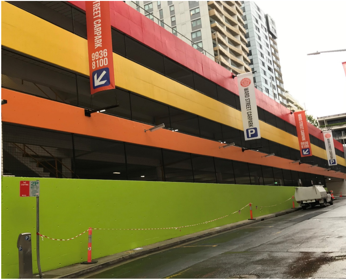
Ward Street Car Park external repainting
