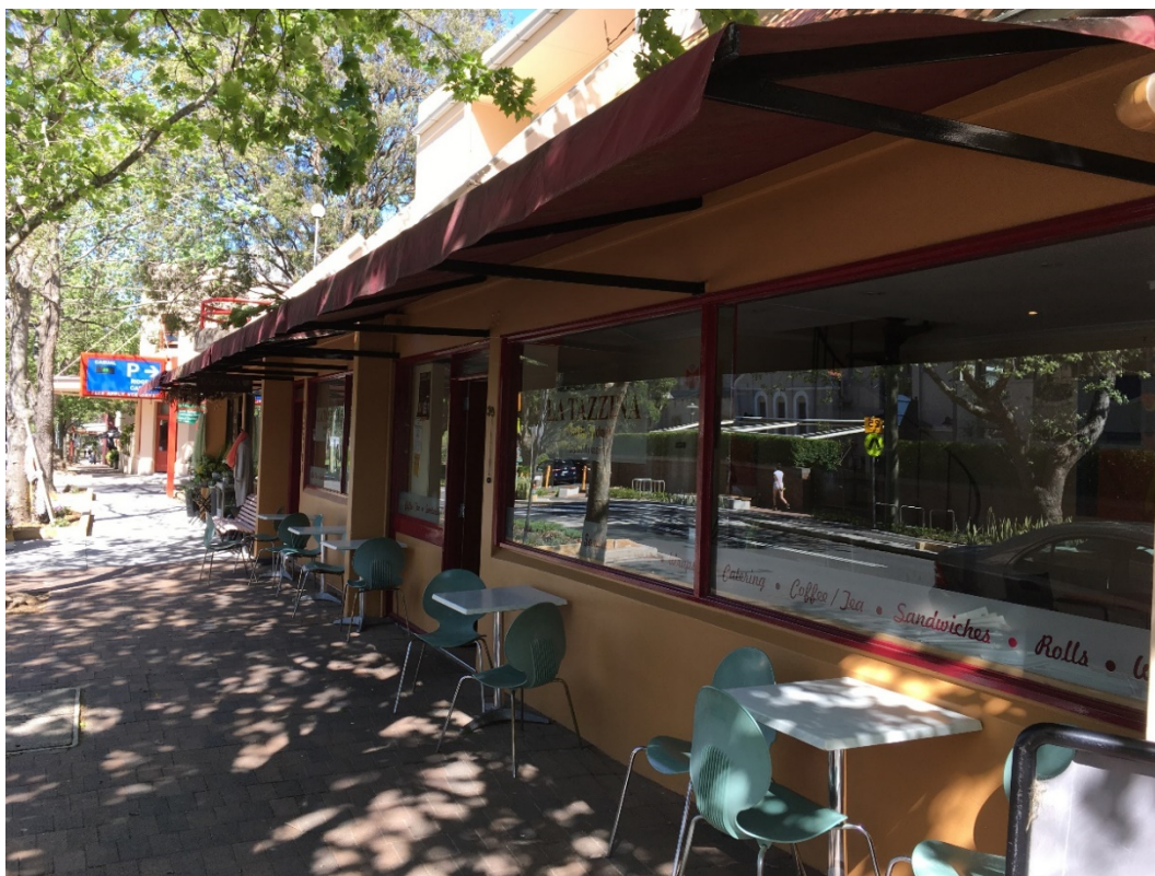
35-41 Ridge Street External repainting
