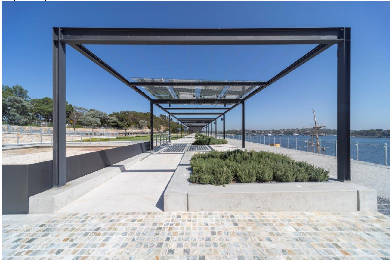
Shade colonnade looking south from northern end showing support wires for grape vines and PV solar & shade canopies
