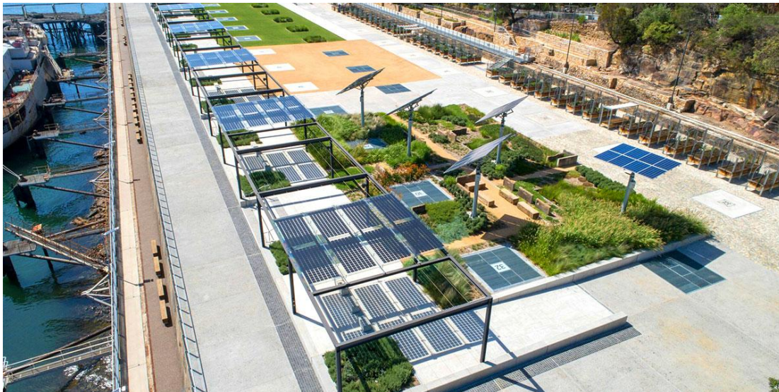
Oblique aerial view looking north showing western shade colonnade with solar PV shade & shelter canopies
