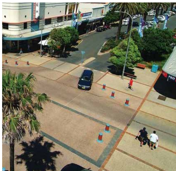
Figure 27 - This table top junction in Port Macquarie, NSW, slows down vehicles and prioritises pedestrians. Intersection improvements within Neutral Bay should consider a similar approach.
