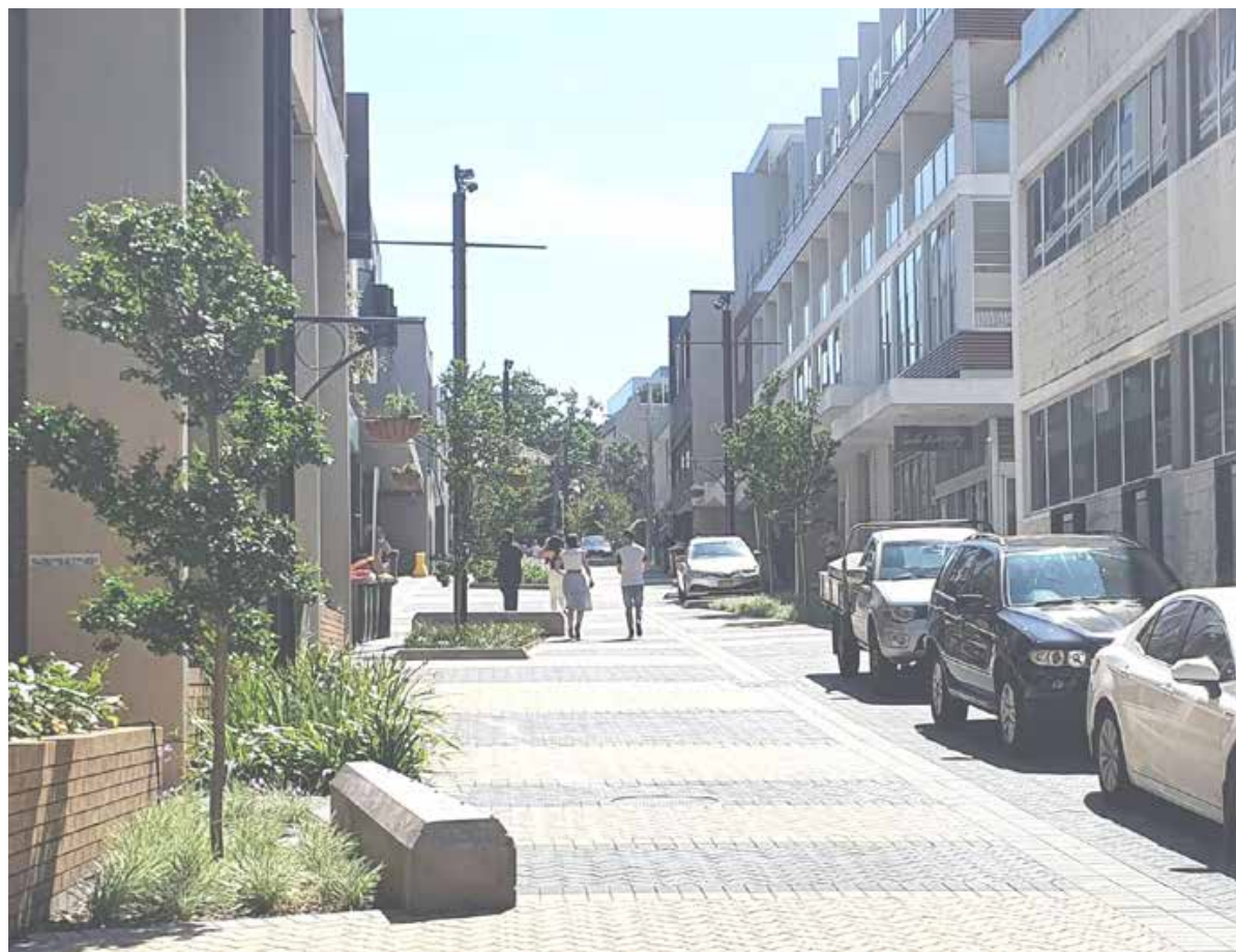
Figure 26 - The recent completion of the Grosvenor Lane shared includes new paving, furniture, landscaping and night-time safety improvements including new lighting. A shared zone enhances the pedestrian amenity significantly as drivers must give way to pedestrians at all times.
