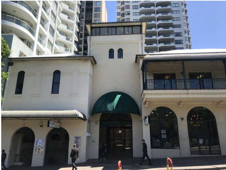
Figure 11 Adjoining building to the south
