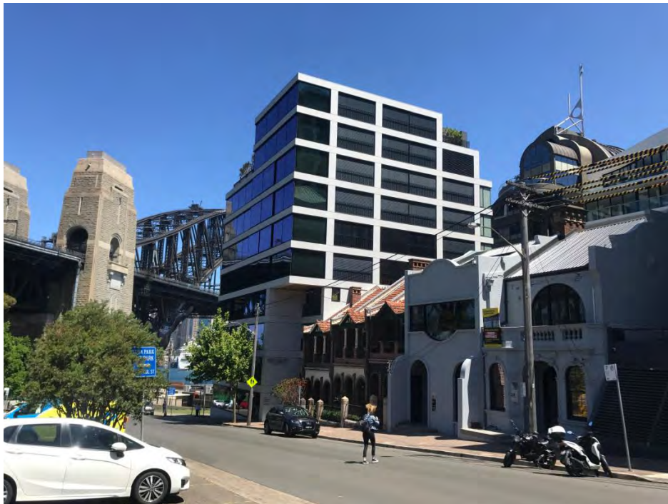
Figure 12 Residential terrace houses and building contained within 20 Alfred Street
