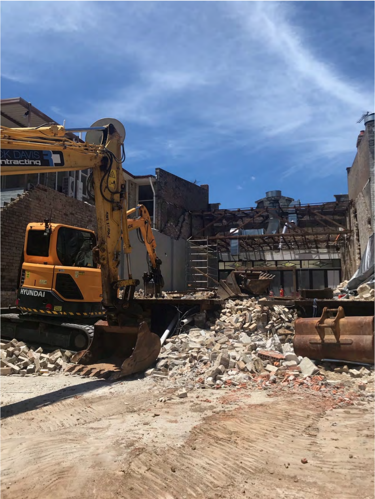
Demolition works in progress 90-92 Willoughby Road
