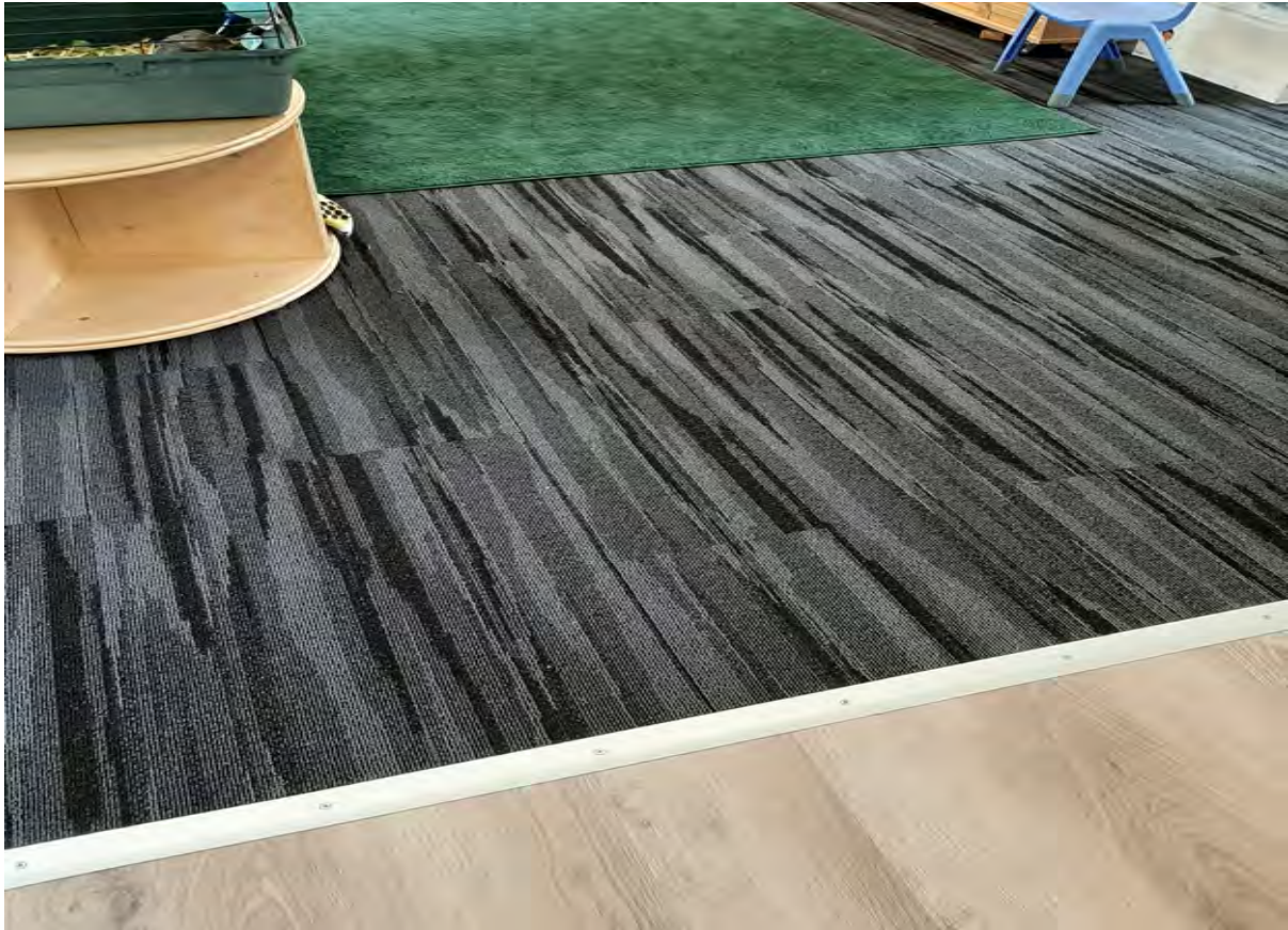
McMahons Point Community Centre Preschool new floor coverings – carpet
