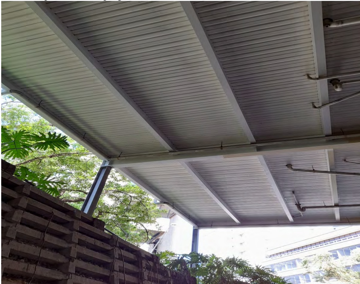
Hume St Car Park 1 Re-Painting
