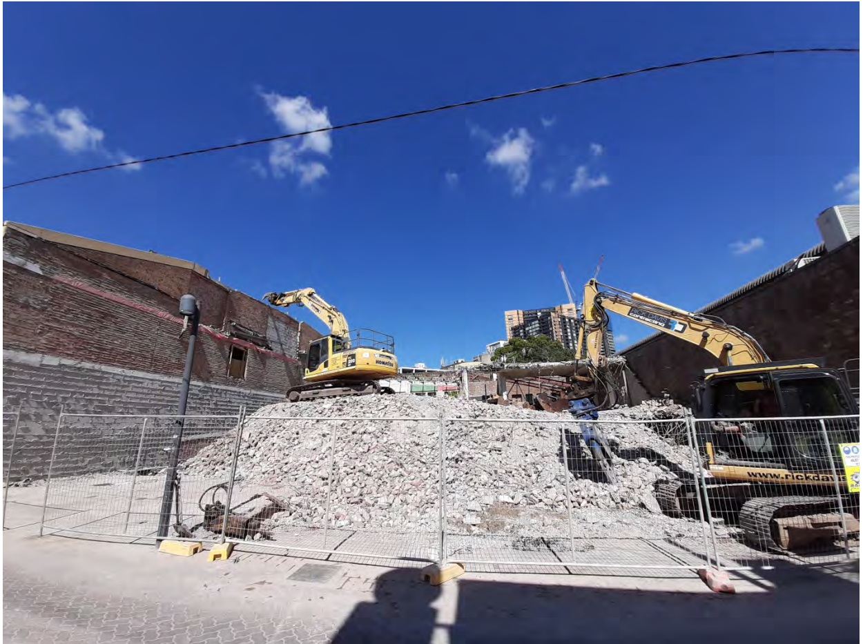
Demolition works in progress 43-49 Hume Street.
