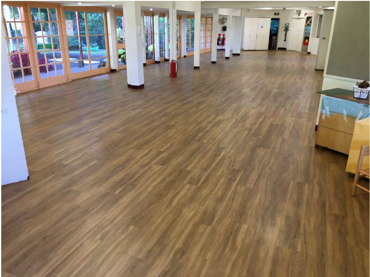
Forsyth Park Community Centre new vinyl planking floor covering
