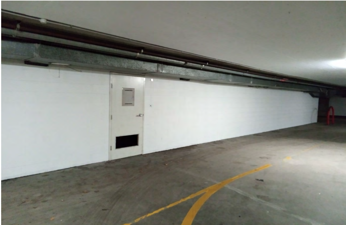
Hume St Car Park 2 Re-Painting
