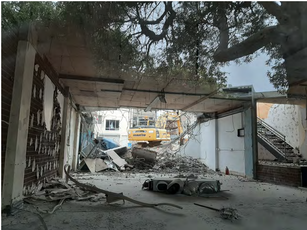
49 Hume Street demolition in progress
