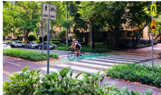
Figure 1: Raised pedestrian crossing, Bourke Street, Sydney.
