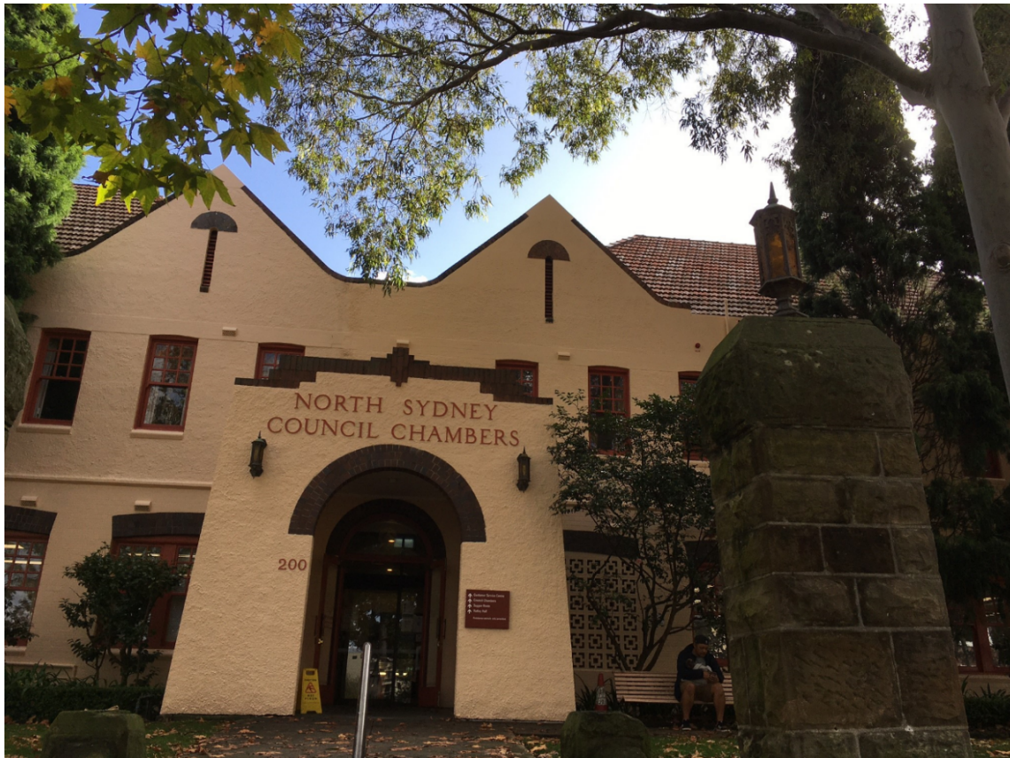
Council Chambers – External repainting on Miller Street frontage
