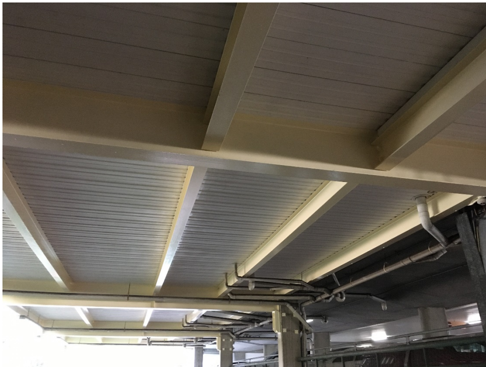
Hume Street Car Park – repainting of steel structural members
