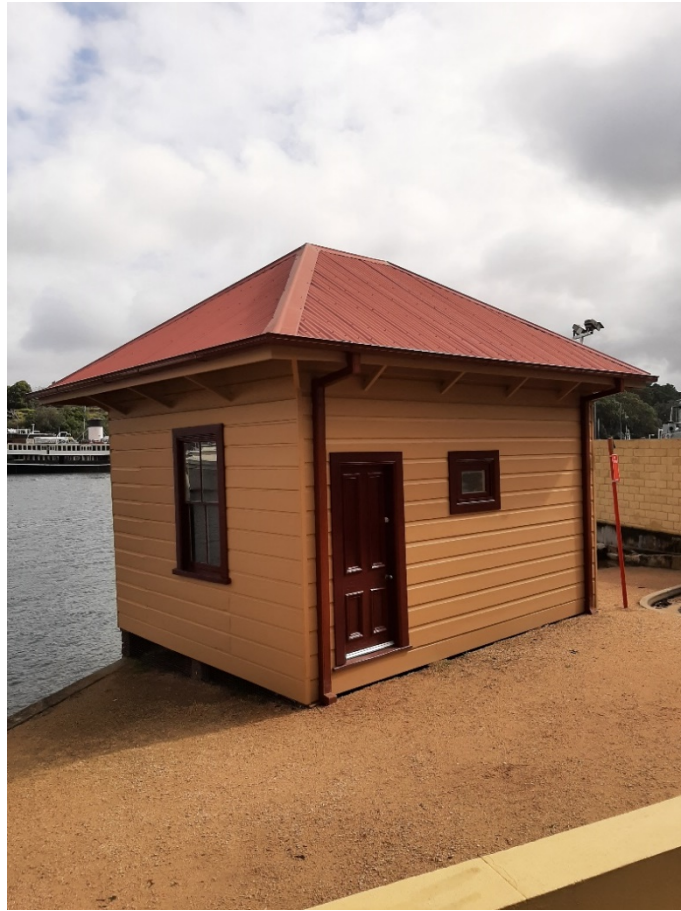
Munro Street Shed after re-painting
