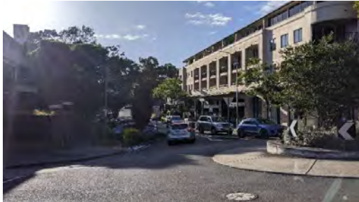
Figure 2.12: Grosvenor Street (looking east)
