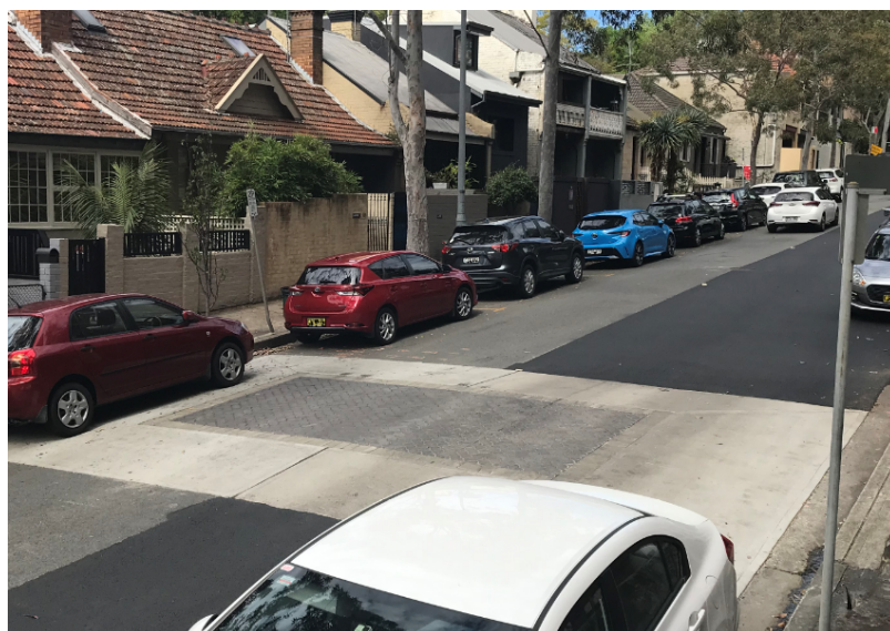
Figure 13. Example of raised flat top threshold.
