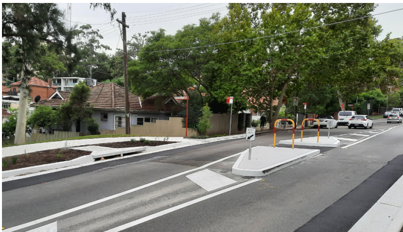
Figure 4. Example of pedestrian refuge to current standards/. A similar level of pedestrian protection is proposed for Kurraba Road
