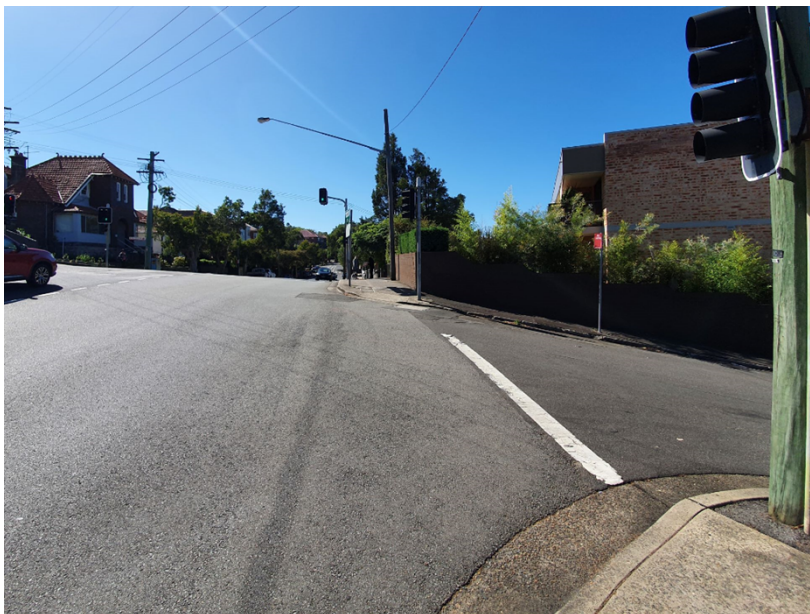
Figure 5. Missing pedestrian crossing facilities at the intersection between Ben Boyd Road and Kurraba Road
