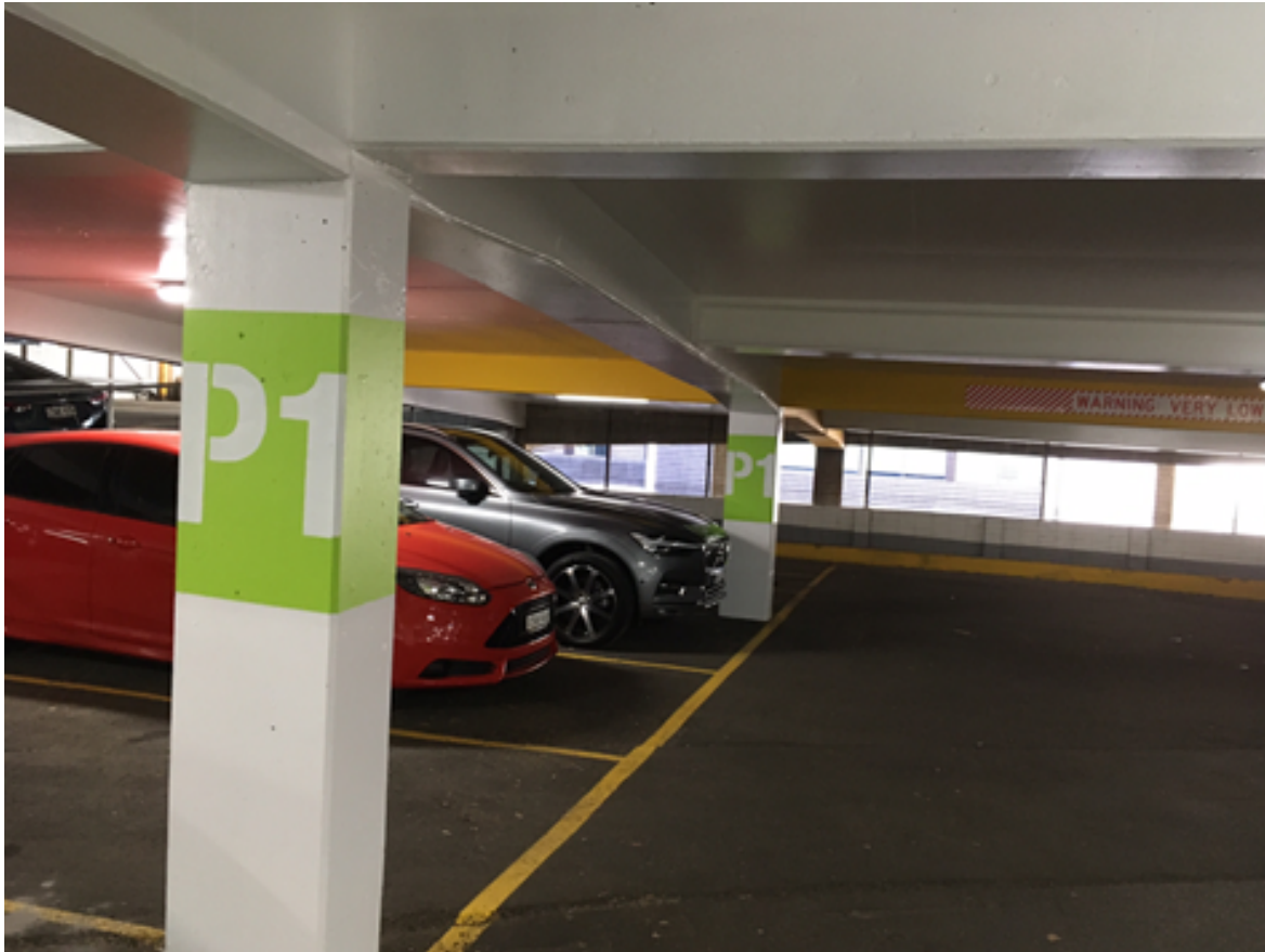
Ward Street Car Park – P1 level signage
