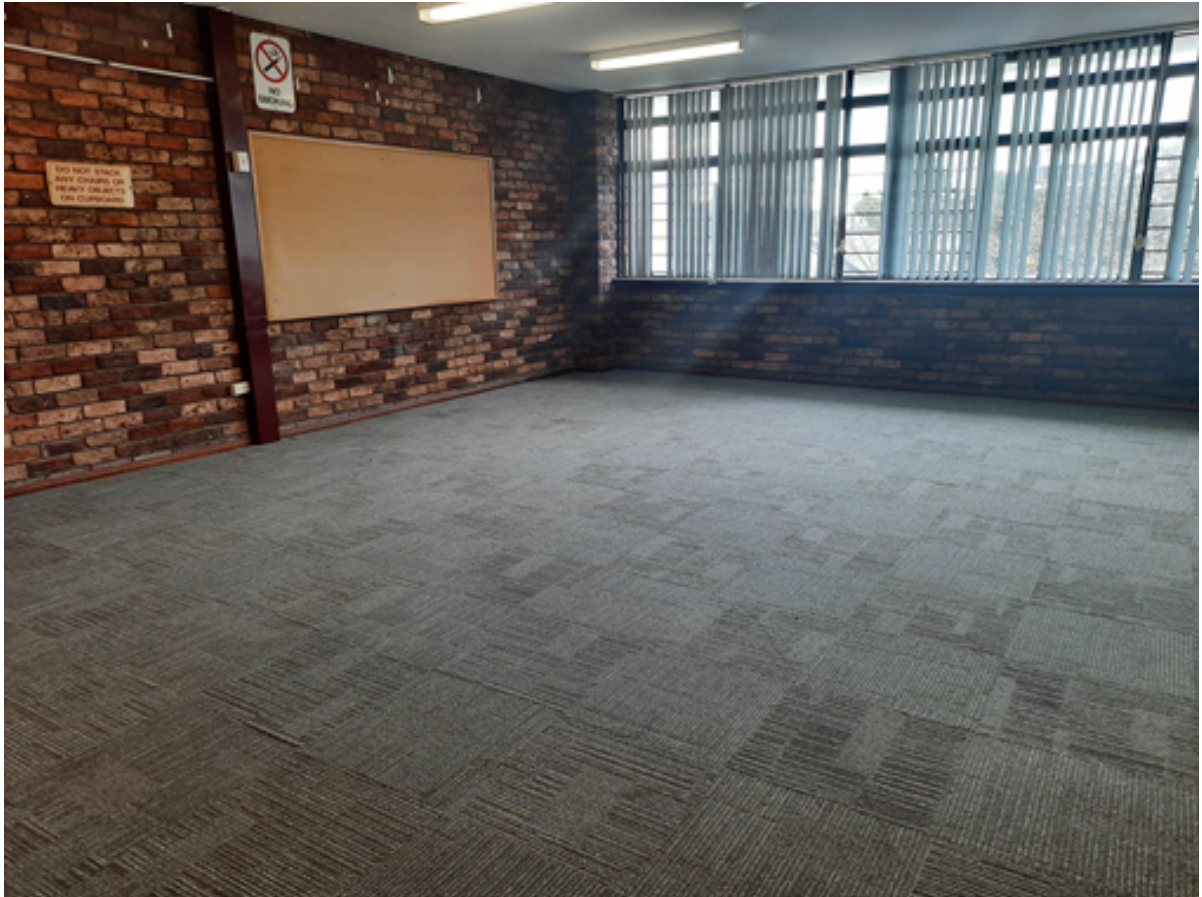
Neutral Bay Community Centre – internal repainting in progress
