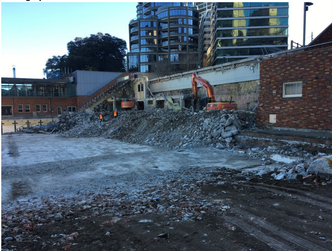
Grandstand removed 06 August 2021
