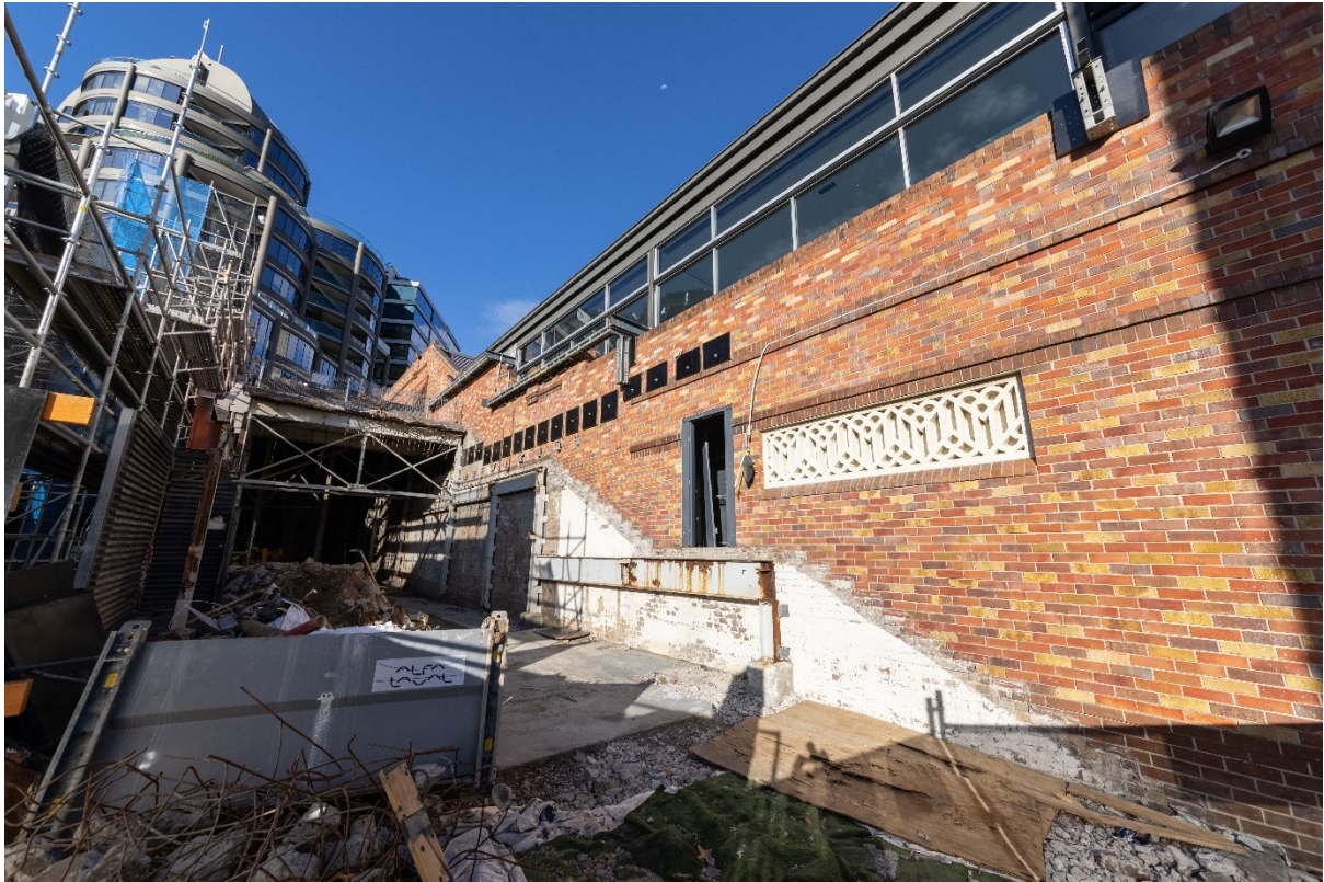
Western Stairs 15 September 2021
