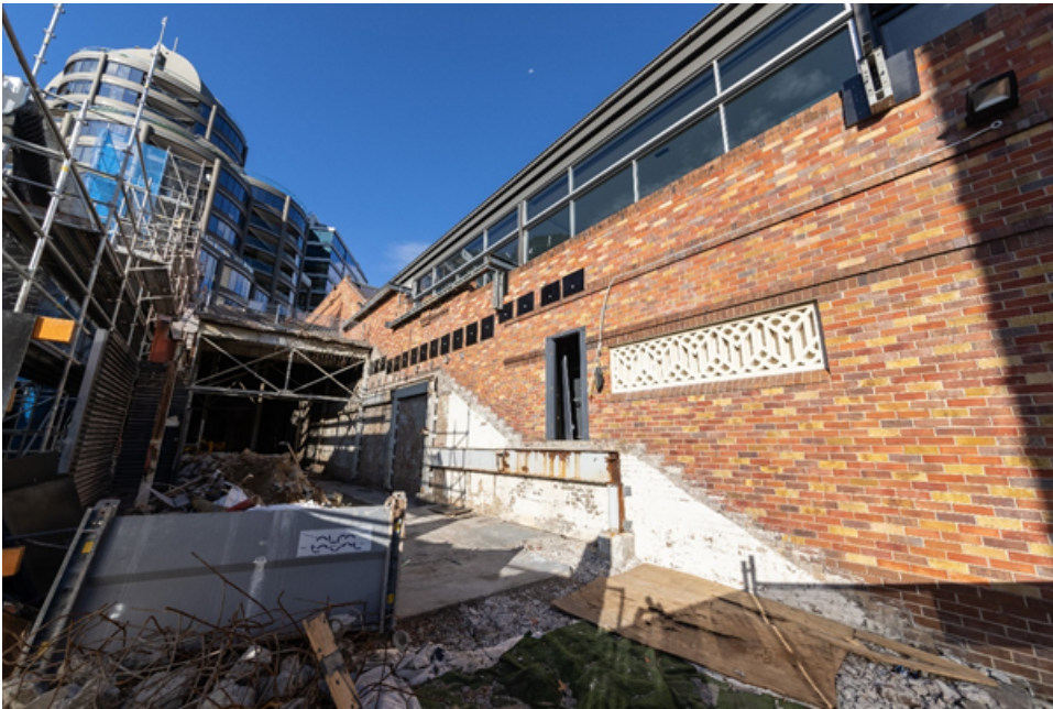
Western Stairs 15 September 2021
