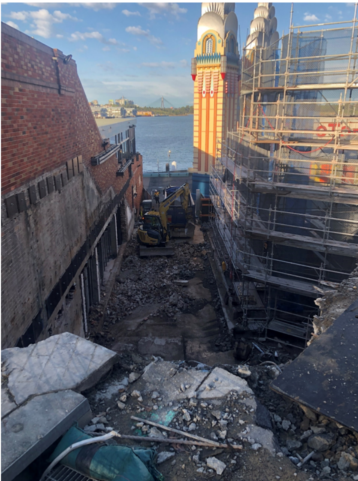
Western Stairs 15 October 2021
