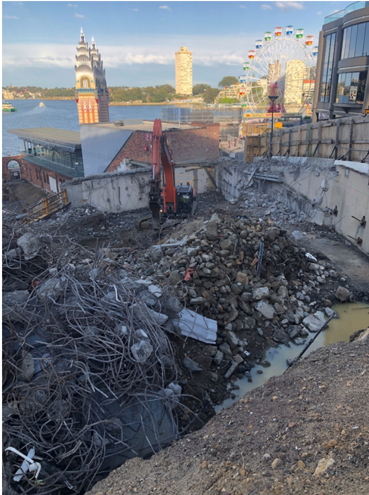
The last of the demolition
