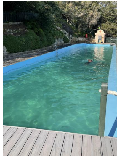
Maccallum Pool - New fencing, decking and pool has been repainted
