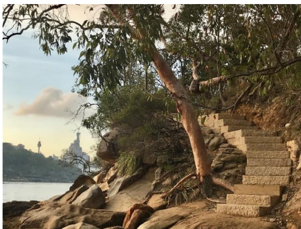
New sandstone stairs to the foreshore
