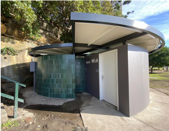
Amenities block – Blues Point Reserve, McMahon's Point
