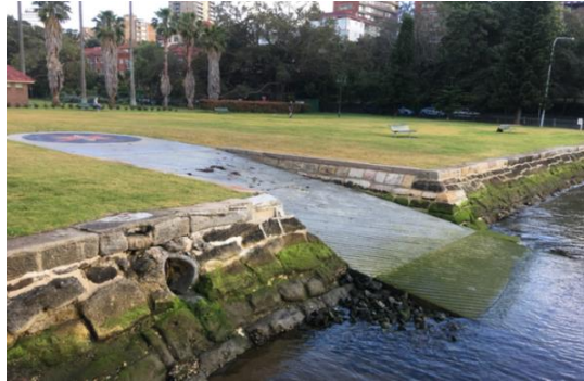
Milson Park boat ramp is now longer, wider and the slope is less steep
